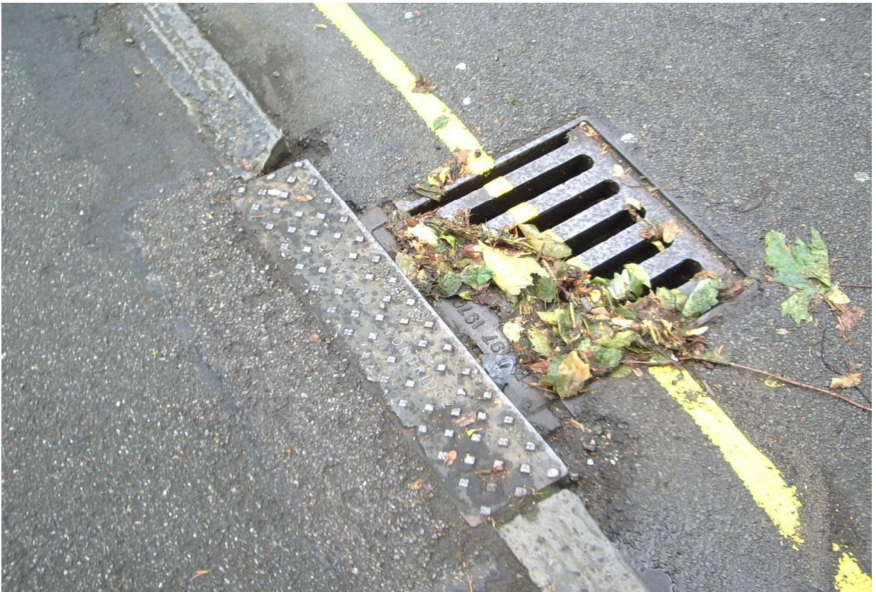
Attractive cast iron street furniture and poorly maintained ragstone kerbs in Hollybush Lane
