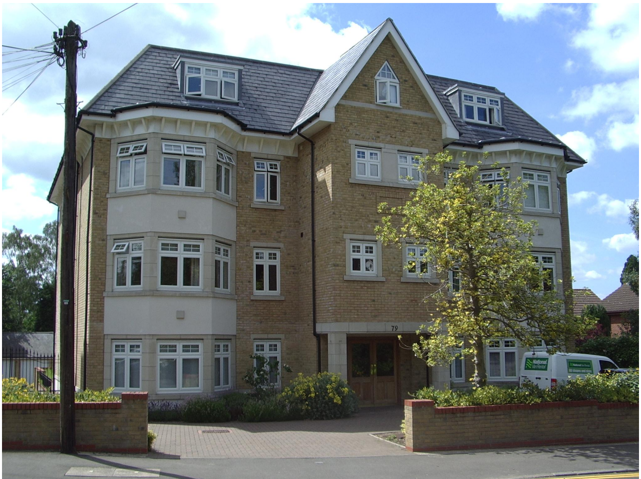
79 Dartford Road on the west side of Dartford Road outside the Conservation Area
