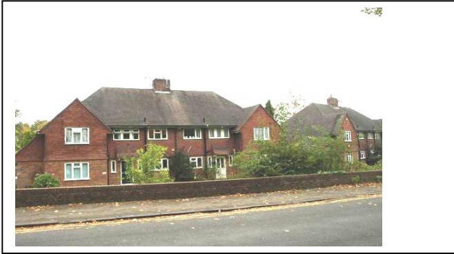
A short row of 1950s houses is arranged in a shallow curve at the north eastern end of the road. The planned row of symmetrically designed red brick and tiled semi-detached houses with hipped roofs and projecting gables forms a unified group.
