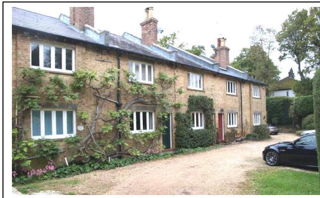
This Victorian row of stone cottages is set back from the road behind a hedge and is not prominent in the street scene. The flat stone front façade, repeated window and door openings, slate roof and chimneys gives unity to the group and acts as a reminder of the origins of the character area.
