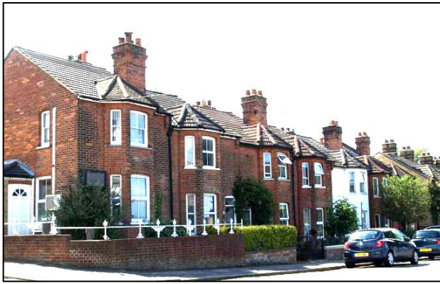
The first seven houses in Gordon Road are excluded from the Granville and Eardley Road Conservation Area. The red brick terraced houses with two storey canted bays on a regular building line form an attractive group and are important to the setting of the Conservation Area. Original windows, doors and roofs have been replaced but decorative chimneys are a consistent feature in the street. A decorative metal railing encloses the corner front garden.
