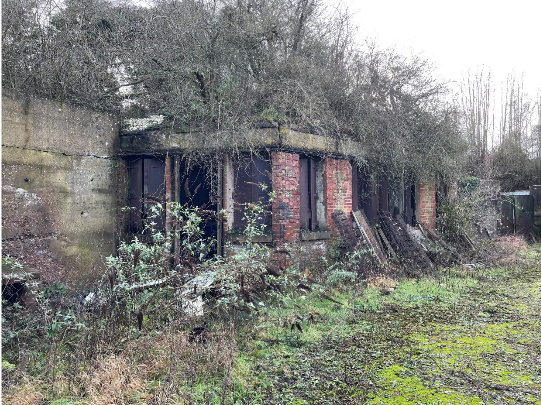
Plate 2 Looking south to the Casemates, with flanking concrete compound wall, and gates thereinto to the south (right)
