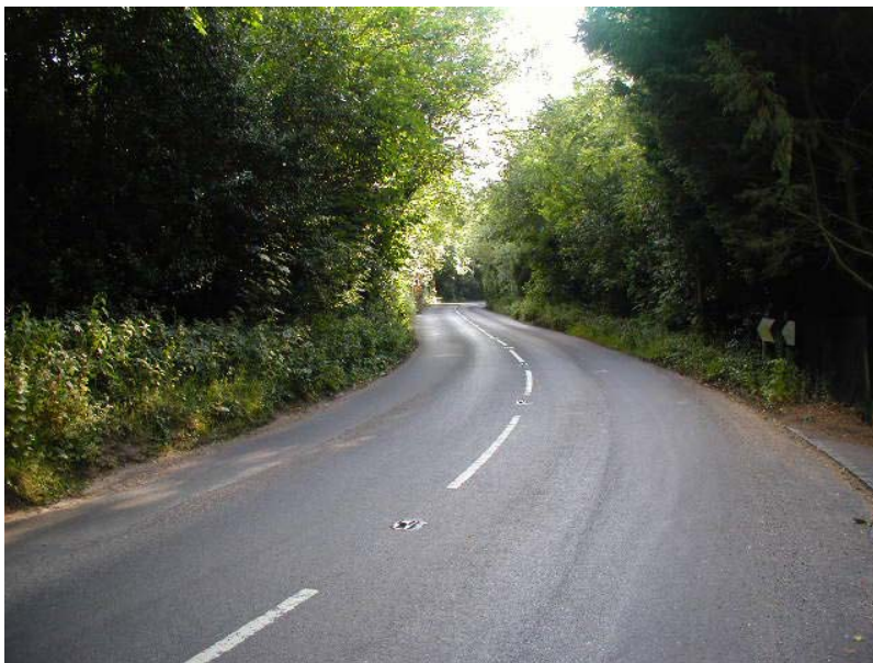
37. Rural scene in Blackhall Lane
