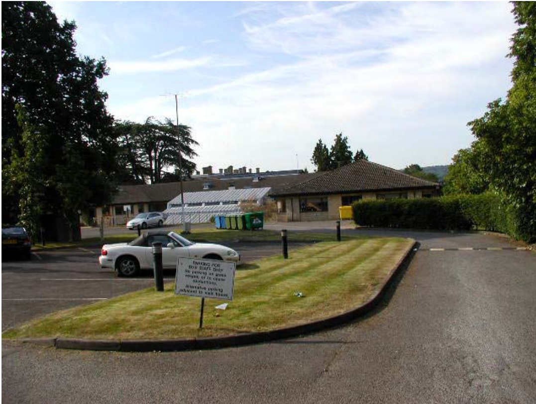
34. This area adjoining Dorton House (Dorton Drive within the Conservation Area) is bland and stark with little planting reflecting the character of the historic area. Also note inappropriate concrete kerbs, where there is a prevalent character and lack of kerbs throughout much of the Conservation Area.
