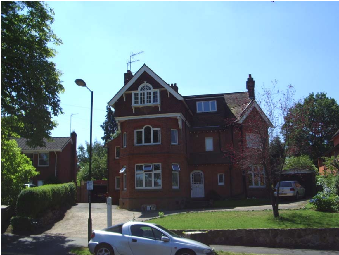
Poor UPVC windows in flats in St Botolph's Road – these require planning permission.
