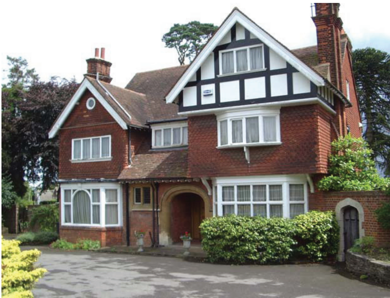
1 Knole Paddock, Seal Hollow Road (This is an example of a quality Edwardian villa it is an interesting and visually important property.)
