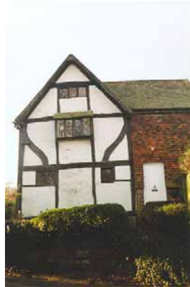
Figure 7 Timber framing 94 Church Road
