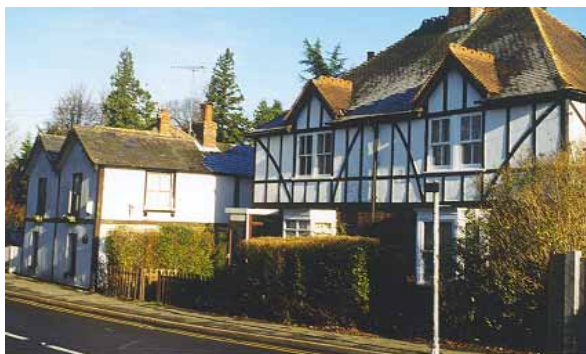
Figure 13 Cottages in Chevening Road
