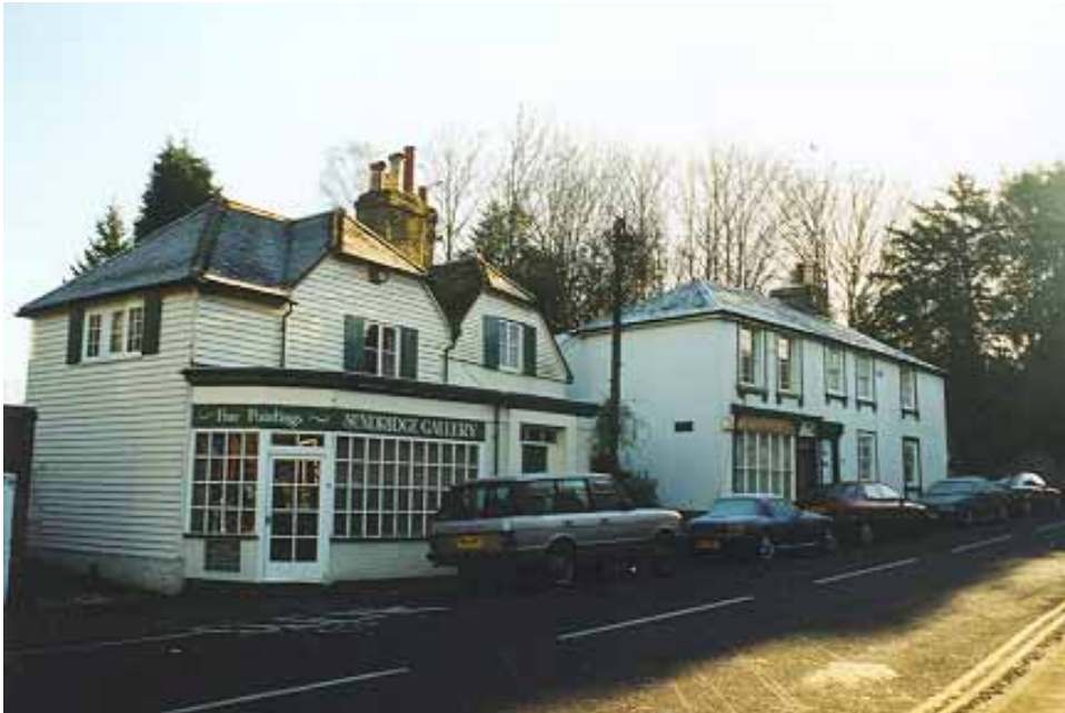
Figure 9 Weatherboarding and shutters on No. 11 Church Road
