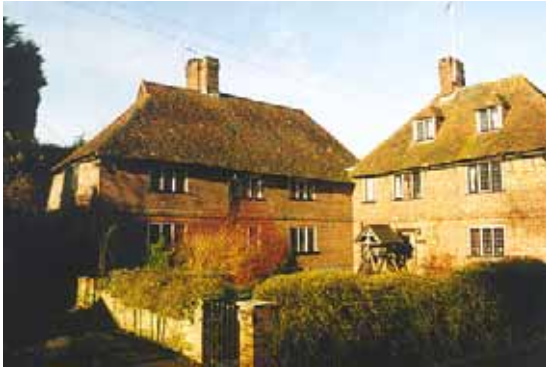
Figure 6 Brick and tile hanging on Well Cottage
