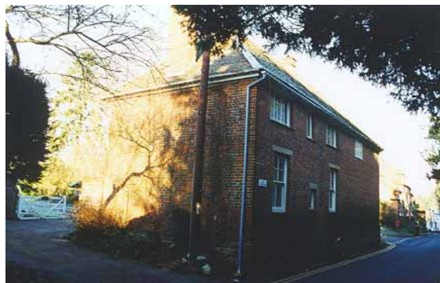
Figure 17 The Gate House, 40 Church Road
