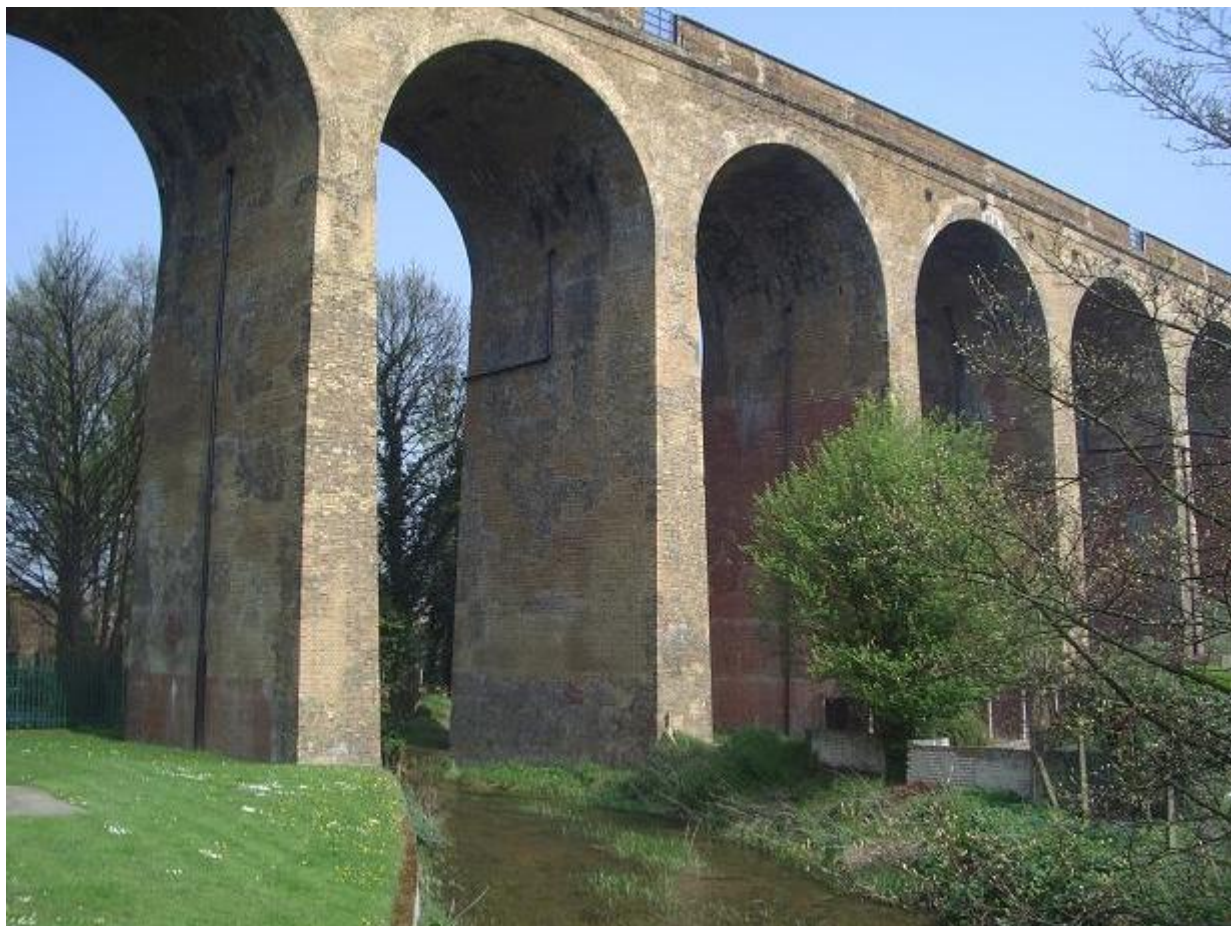
8. The railway viaduct, originally built in 1864 was constructed using yellow stock bricks and has been repaired using inappropriate red bricks. Whilst it is visually separate from the mill it is still an important part of this industrial grouping and makes a significant contribution to the character of the conservation area and together with the mill stack is a dominant feature of South Darenth.
