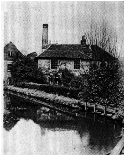
Fig. 2 Mill House in Early 20 th Century
