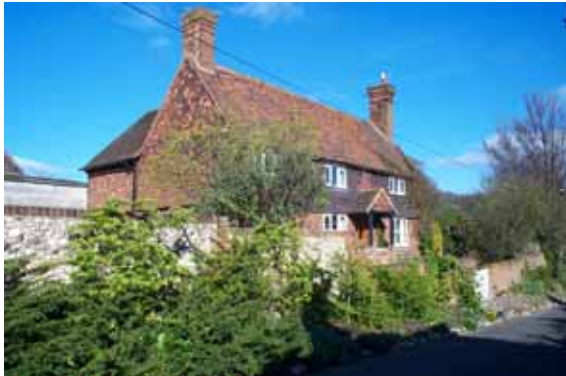
Fig. 1 Oxbourne Farm House
