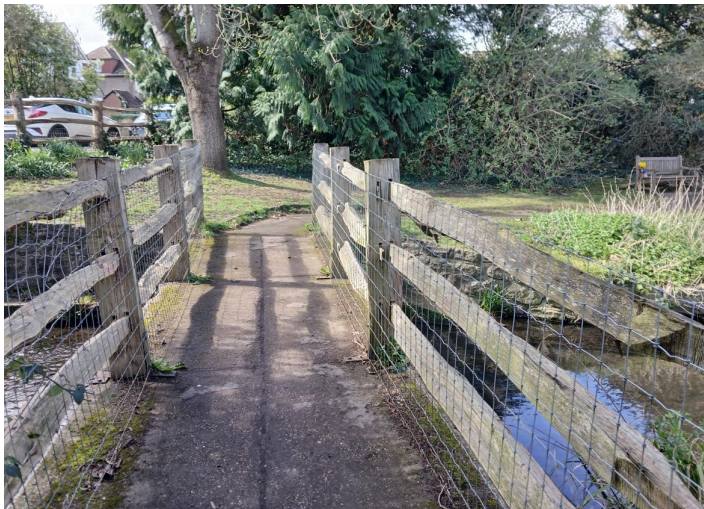
Bridge across the stream – north side, summer
