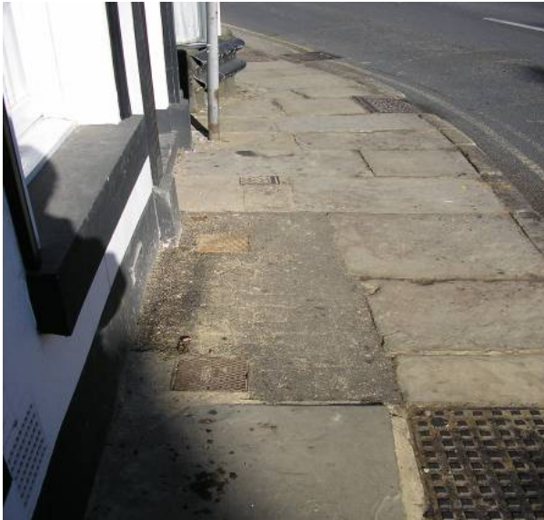
Loss of stone paving and poor quality reinstatement
