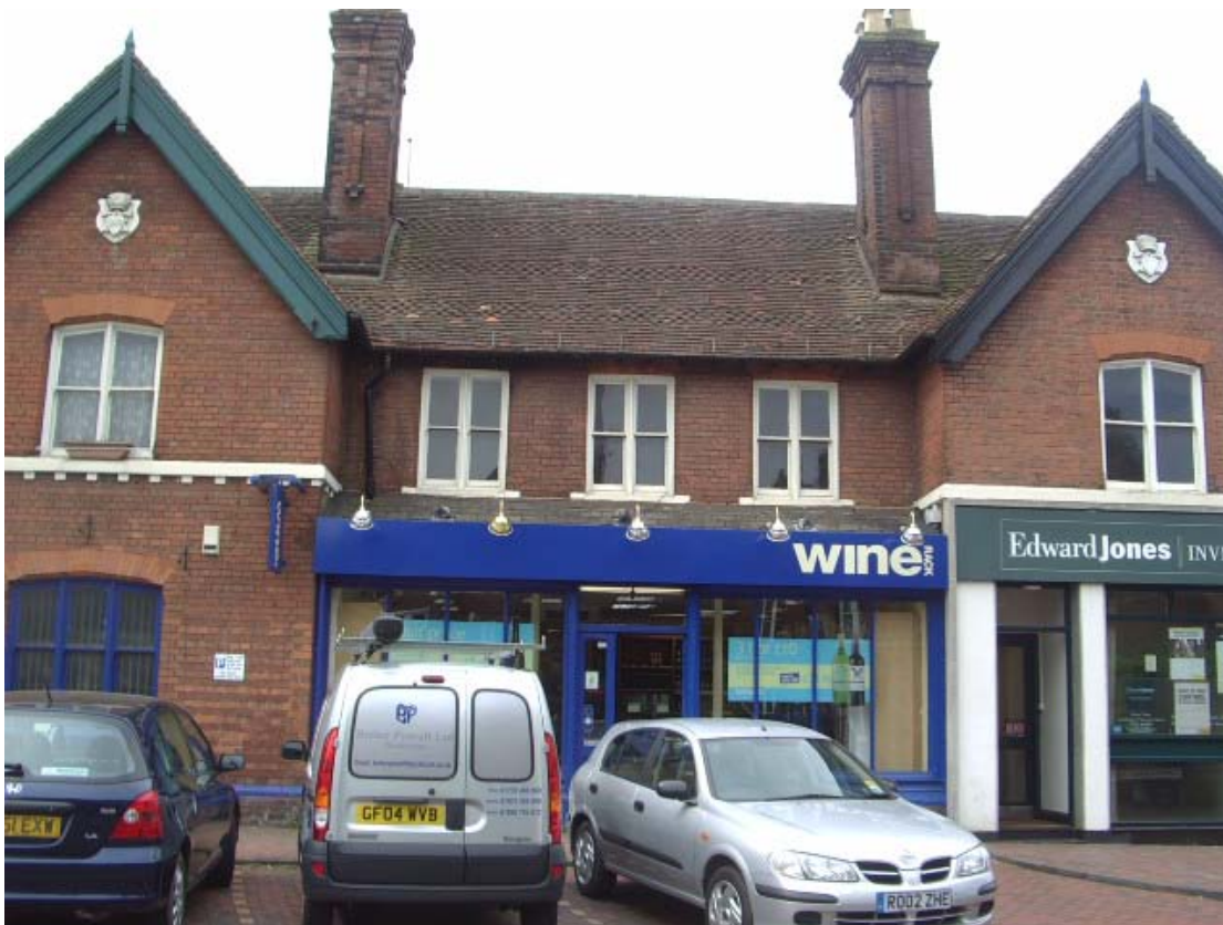
57. Inappropriate shopfront in The Square
