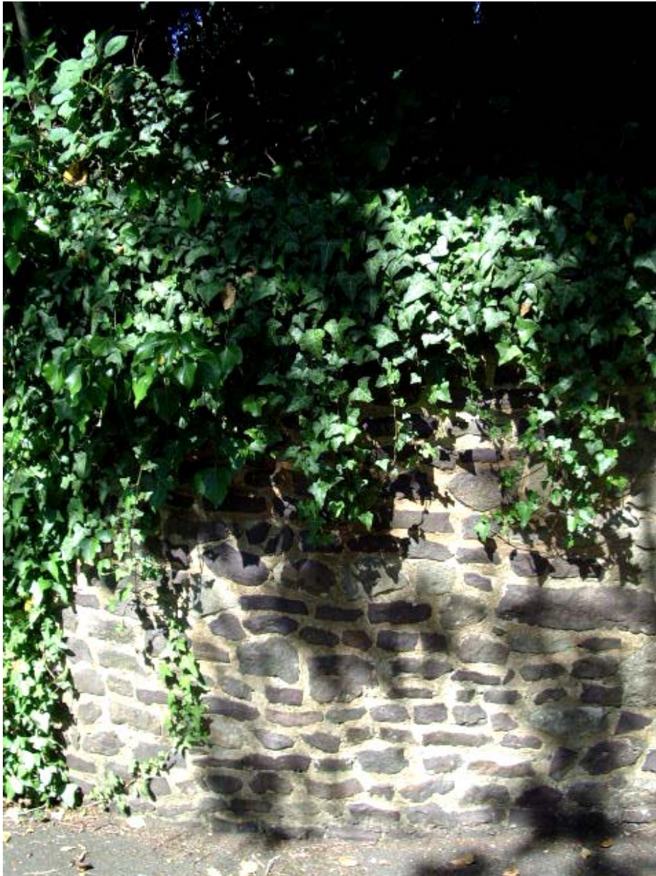
61. Unusual ironstone wall in Shoreham Lane
