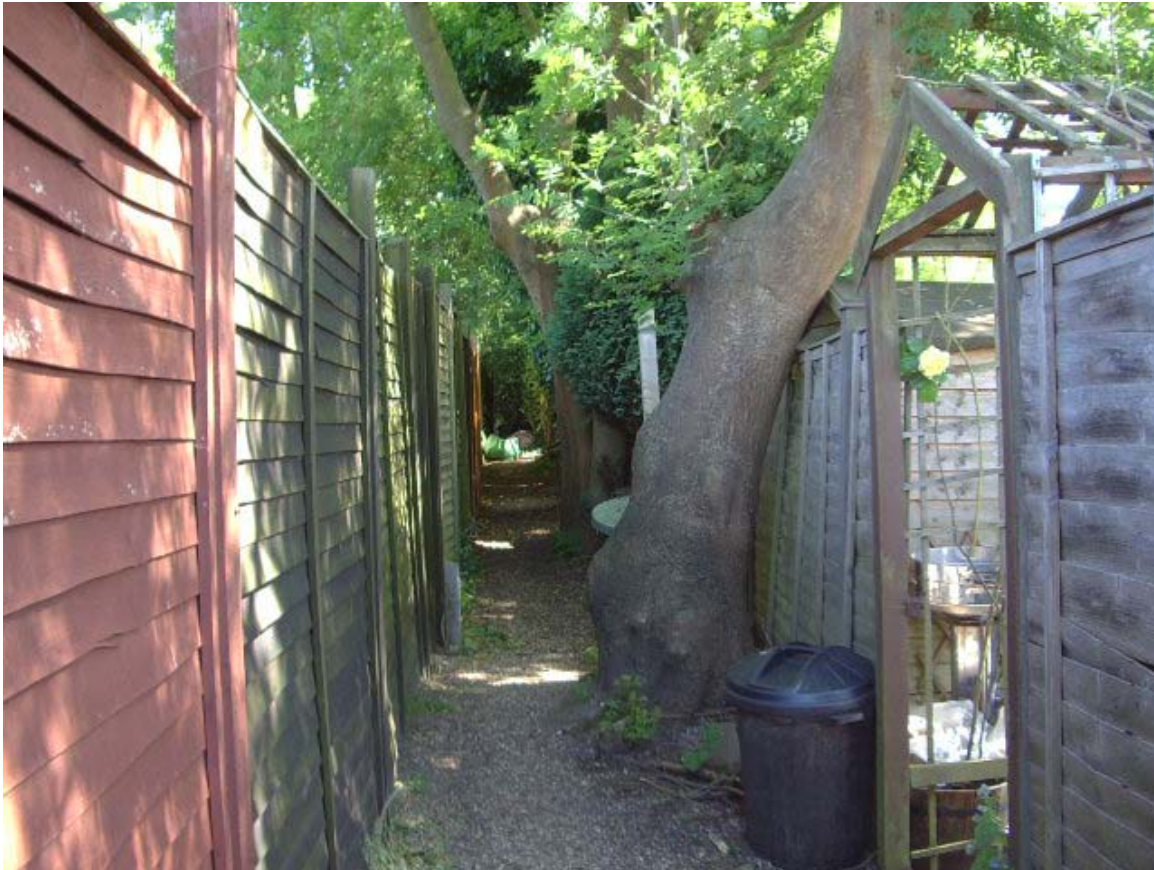
58. Attractive service alley at the rear of cottages on East side of London Road adjacent to St Mary's Church
