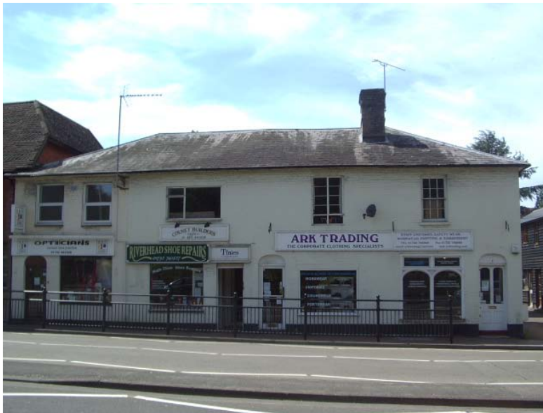
41. In London Road many of the residential properties have been converted to shops, sometimes to the detriment of the original detailing.
