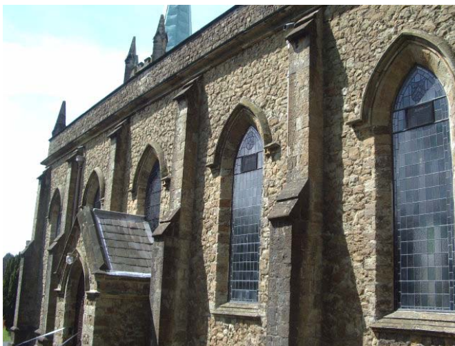
23. The Church of St. Mary stands on high ground dominating the Square. It is built of ragstone and has a copper spire that rises out of the surrounding group of mature trees.
