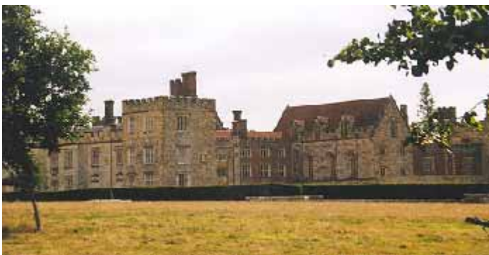
Fig. 27 Penshurst Place from the north
