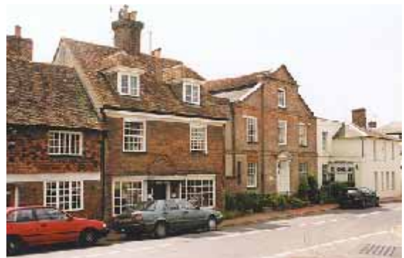
Fig. 6 Variety of roof heights and detail add interest to the street scene
