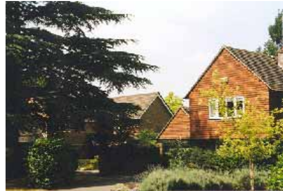
Fig. 34 The new development at Latymers
