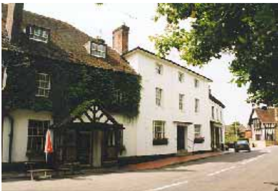
Fig. 15 The view towards the road junction
