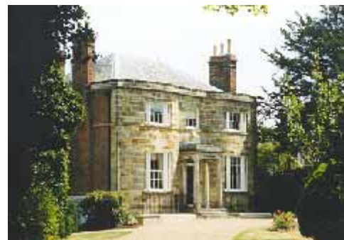
Fig. 11 The Yews adjacent to the bridge over the Medway
