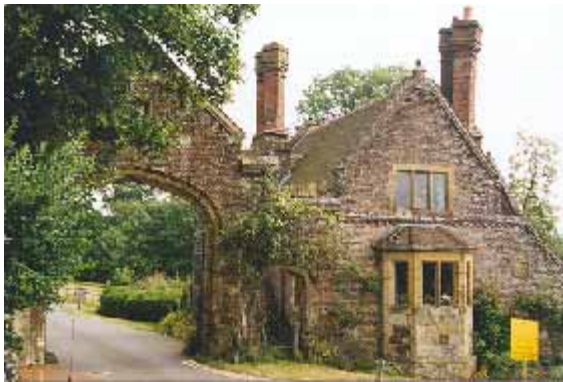
Fig. 13 The Gateway and Lodge to Penshurst Place
