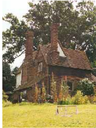
Fig. 42 Thimble Hall Cottage behind the telephone exchange
