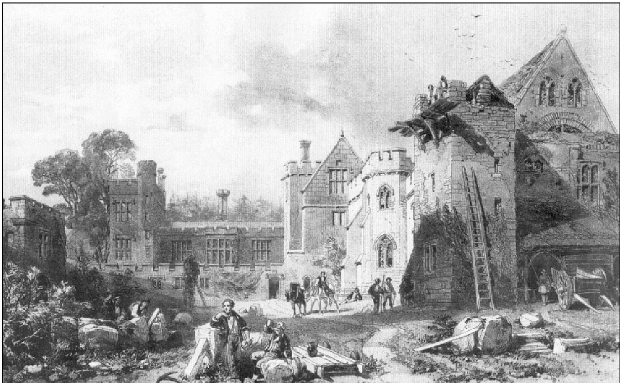
Fig. 3 Restoration work at Penshurst Place in the 1840's
