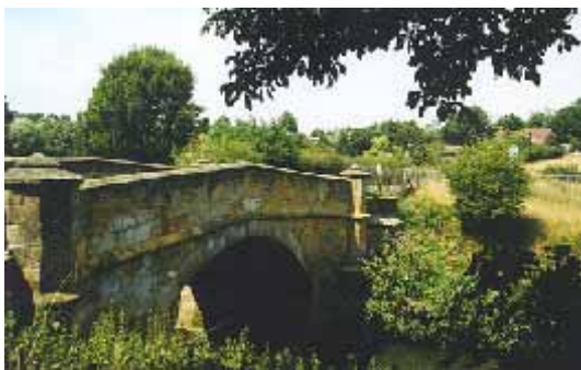
Fig.39 The Medway bridge
