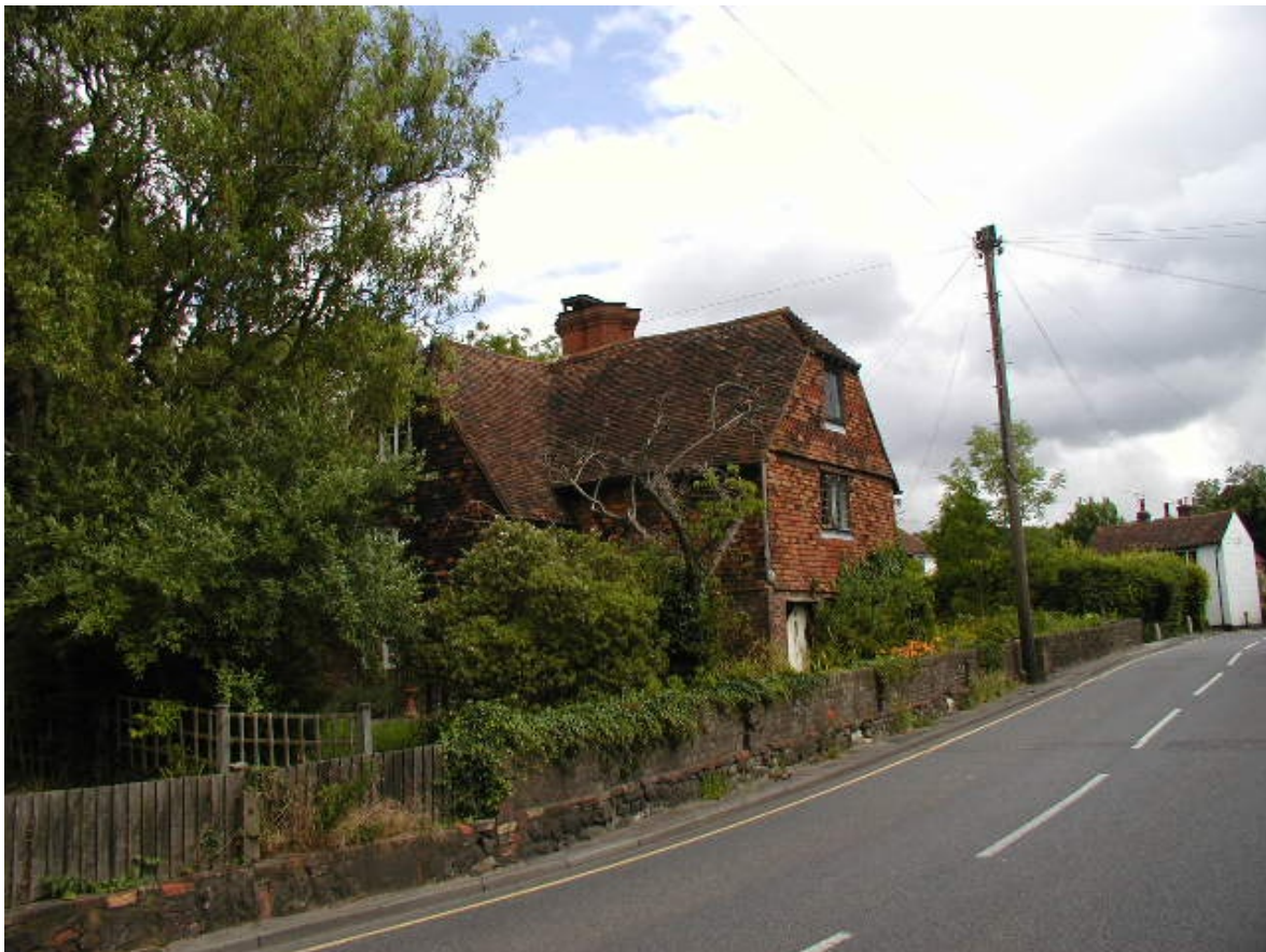
64. Traditional Wealden farmhouse. The warm colouration of locally made brick with tile-hung façade beneath a barn hip roof of hand-made Kent peg tiles. A typical Kentish yeoman's home.
