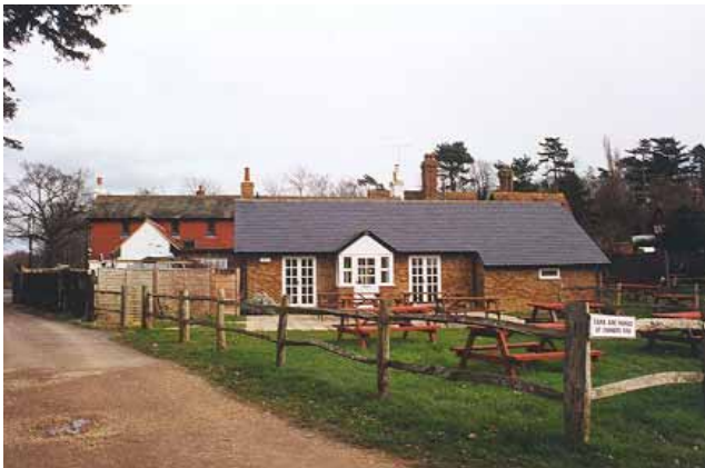
Figure 14 Rear extension to the Kentish Horse
