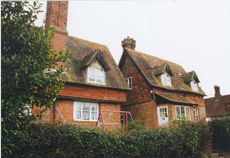
Figure 3 1 - 2 Cow Lane and Markbeech Cottages
