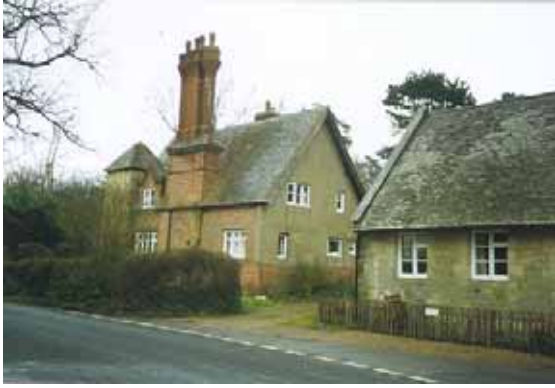
Figure 7 Old School Cottage, School House and The Old School
