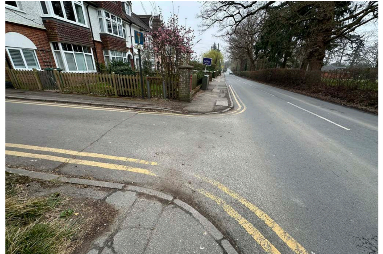
Figure 5.17. Example of poor crossing provision at side road at Mill Hill (LCWIP Route 7).
