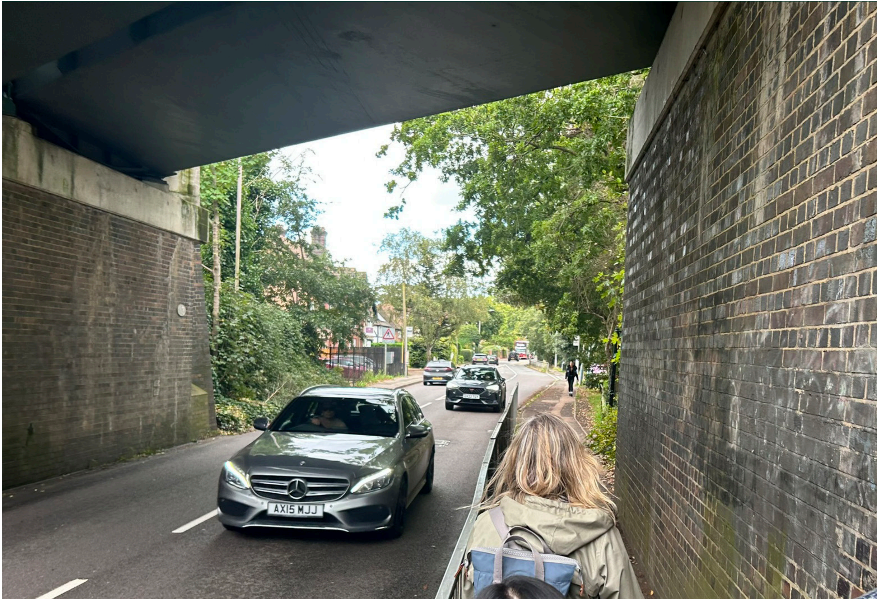
Figure 3.2. Station Road Railway Bridge
