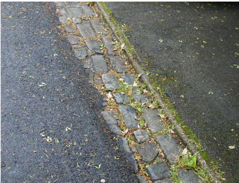
Historic setts in Oakhill Road
