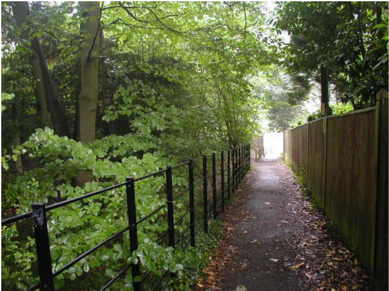
Attractive new railings based on historic designs in the Conservation Area
