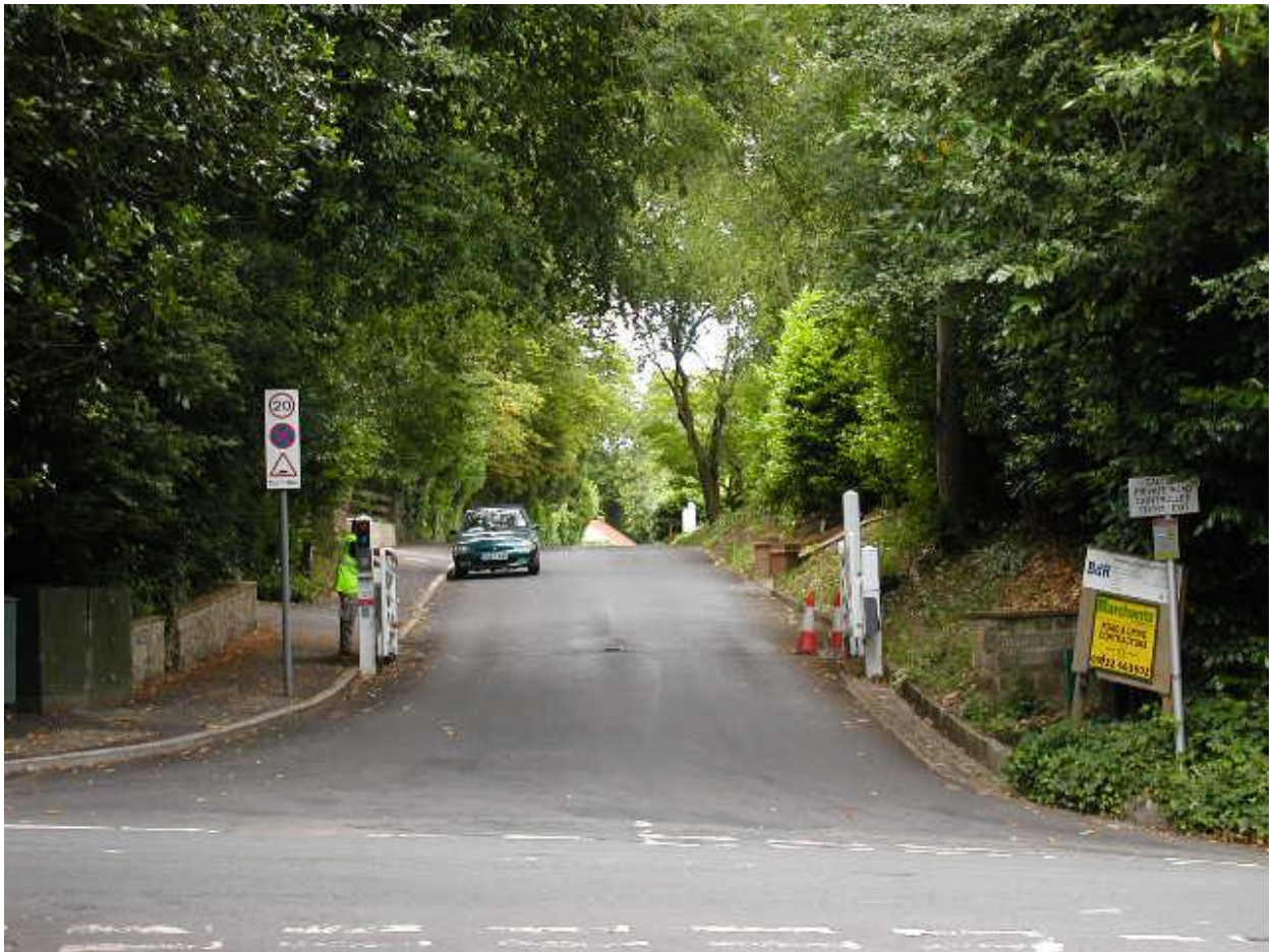
Oakhill Road entrance – compare with simplicity of entrance to Kippington Road
