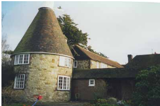
Figure 5 Victorian Oast House (Rondavel)
