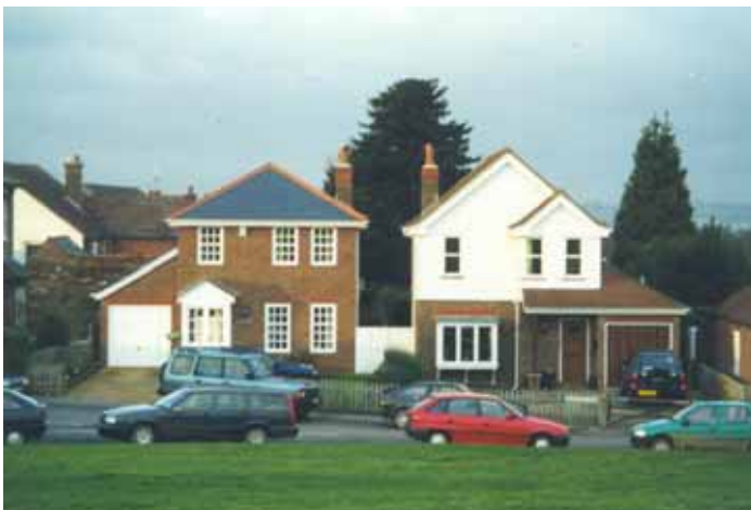
Figure 11 Dove Cottage and Pump House
