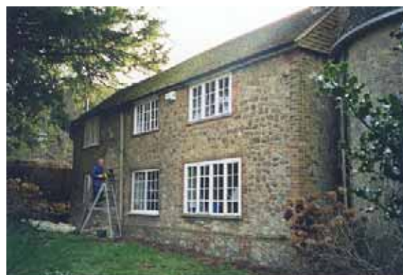
Figure 33 Victorian oasthouse showing repairs/adaptations being carried out
