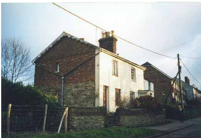
Figure 15 Hope Cottage, Sundridge Road, with rubble and brick boundary wall.
