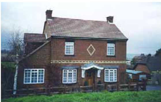
Figure 28 and 29 The detailing of Whitelea contributes to the conservation area
