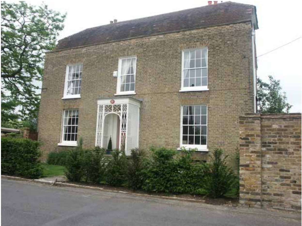
Fig 57: Restored timber porch Croft House, The Street
