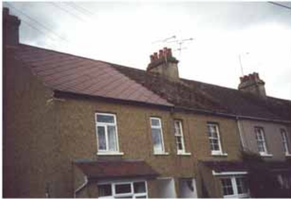
Fig 14: Bexley Cottages, The Street
