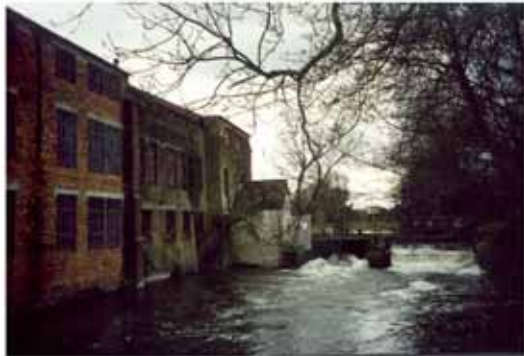
Fig 38: Former view looking south from the bridge
