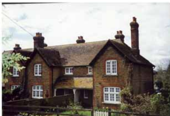
Fig 19: Court Lodge Cottages, Horton Road
