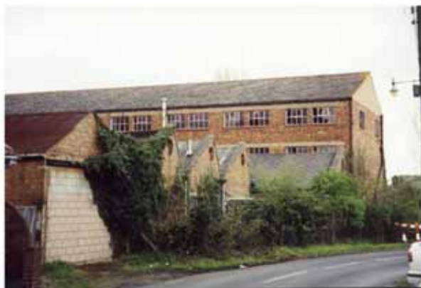
Fig 31: Westminster Mill, before redevelopment.
