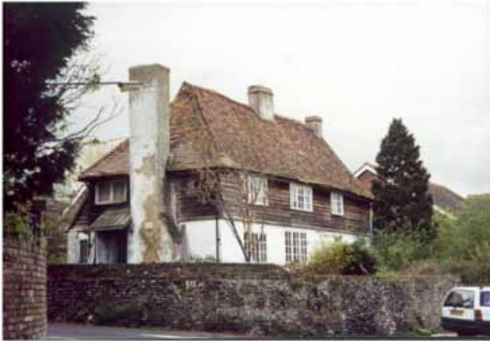
Fig 55: Cement based repairs to chimney stacks, Old School Cottage
