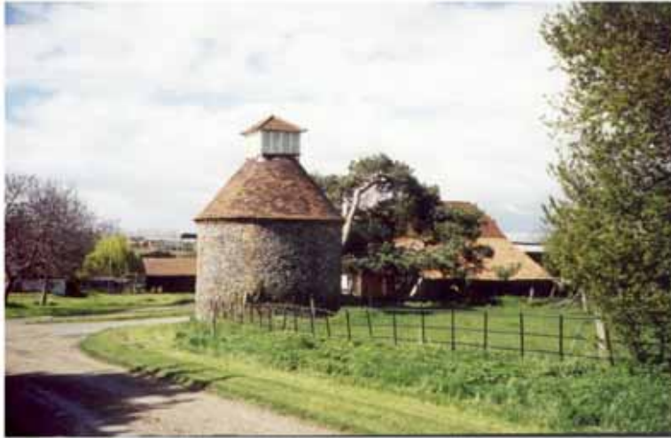
Fig 51: Dovecote and hip roofed barn, Court Lodge Farm.
