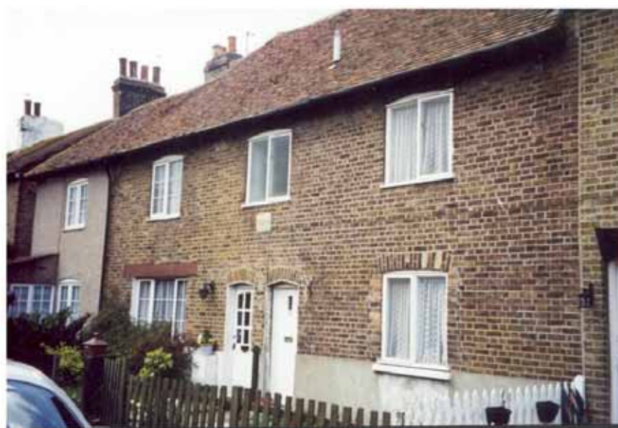
Fig 66: Unsympathetic alteration of window opening
