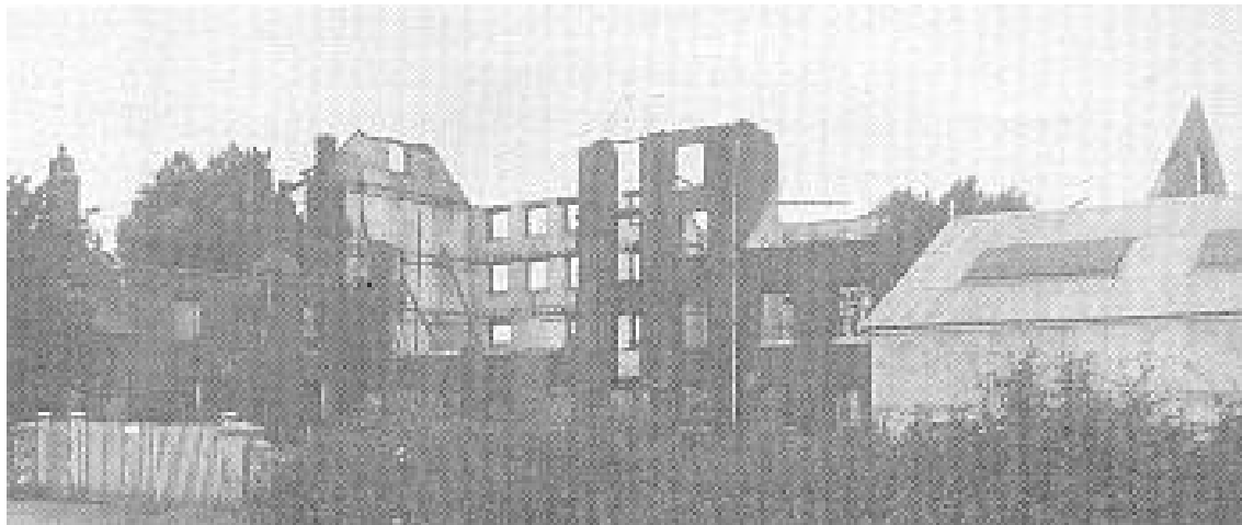
Fig 7 Westminster Mill: Fire caused by lightning.
