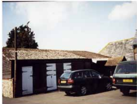
Fig 3: Stable Block, Holywell Farm
