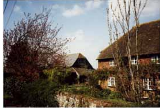
Fig 16: Brick and flint wall, Holywell Farm
