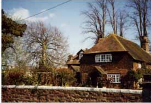
Fig 15: Brick walling with white painted brick capping
