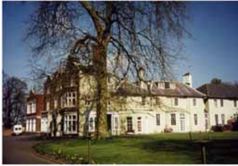
Fig 8: Main building to Holywell Park
