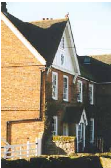
Figure 4 The Manor House
