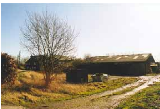
Figure 16 The modern farm buildings behind Walnut Tree Cottage
