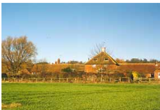
Figure 11 A view north towards the converted farm buildings
