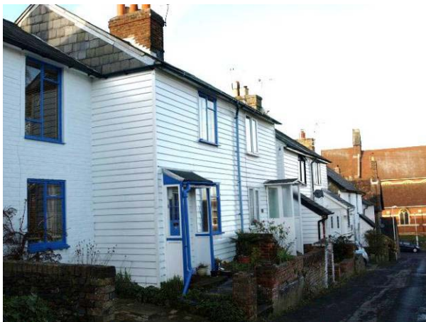
West side of Prospect Road
