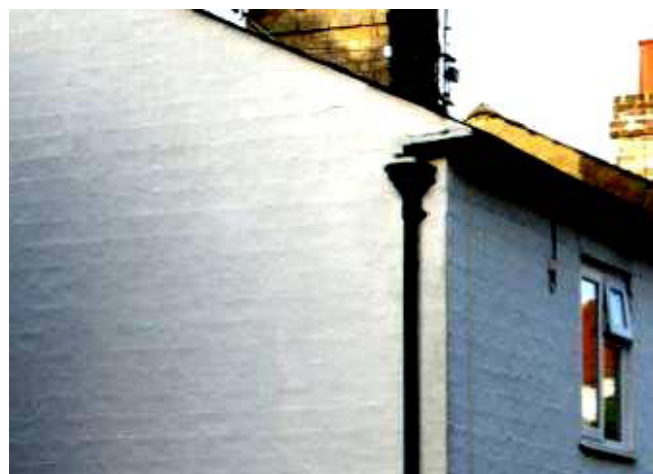
Rat trap brick bonding at 21 Sandy Lane
