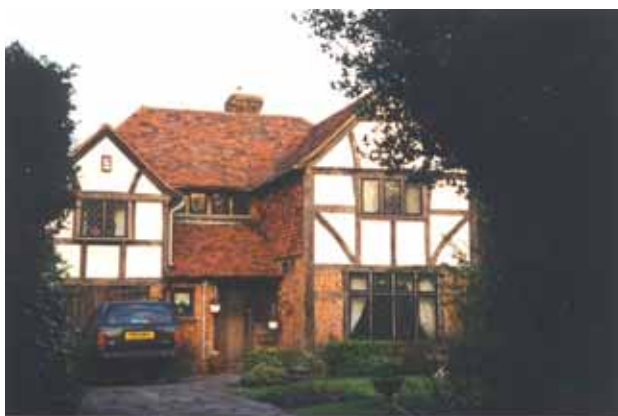
Fig 23: Tudor Cottage, Church Road
