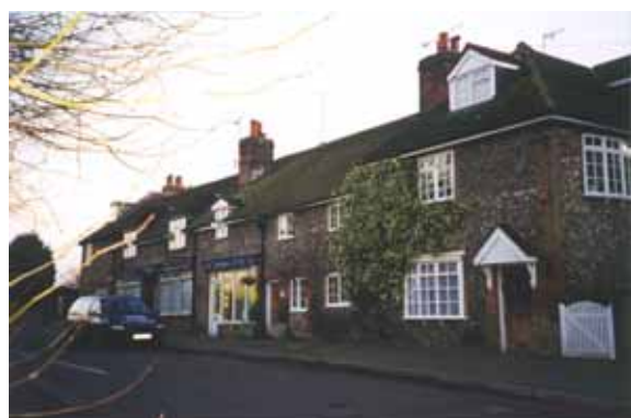
Fig 2: Vernacular architecture using local flint as building material, Church Road
