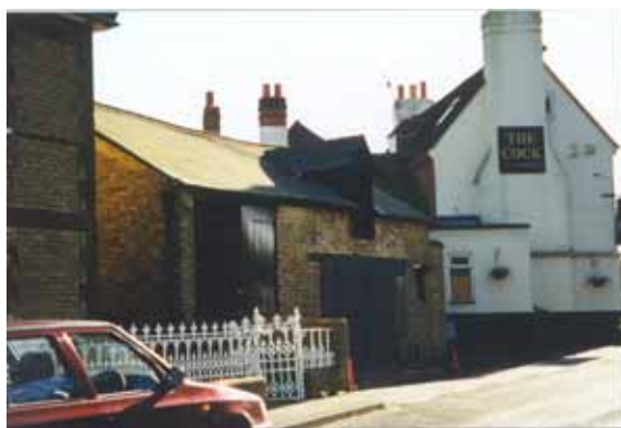
Fig 25: The outbuilding to The Cock, Station Road
