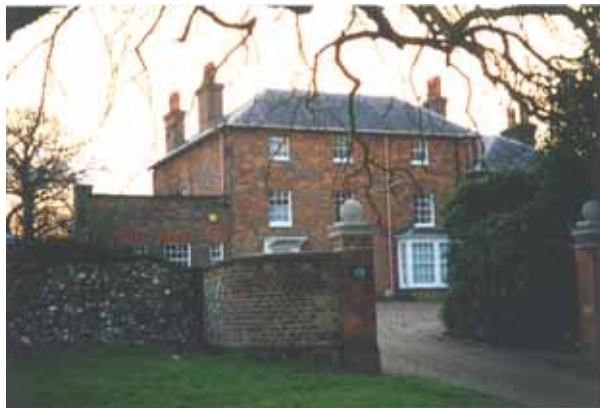
Fig 1: Village House and associated boundary walls, Church Road
