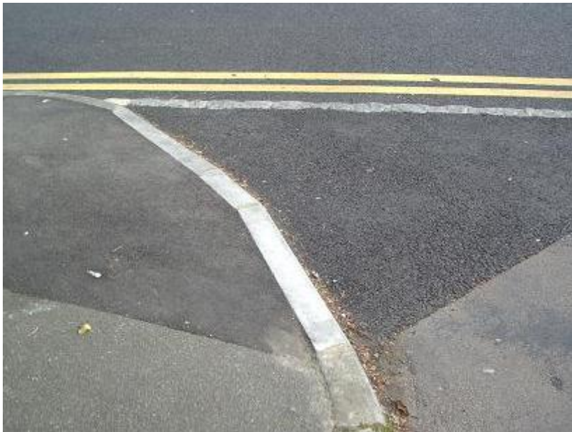
Example of poor highway maintenance South Park - note stone kerbs, concrete kerbs, granite setts and blacktop
