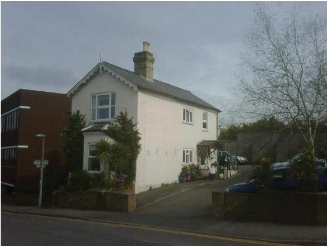
UPVC windows in Argyle Road
