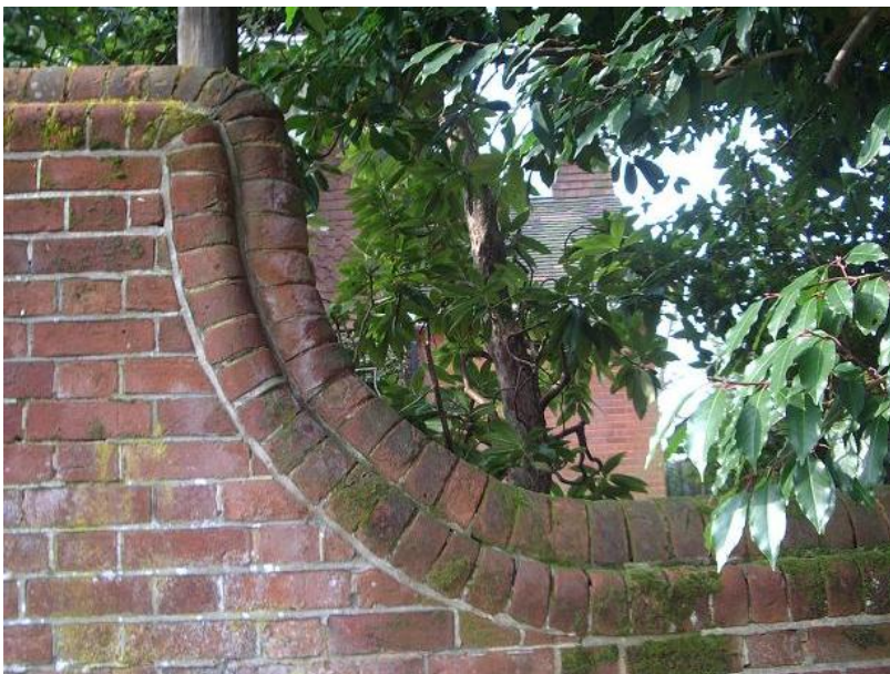
Good wall in South Park
