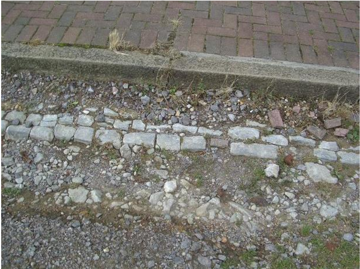
Historic Setts in Clarendon Road
