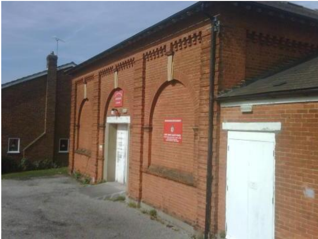
Good brickwork on army cadet building in Argyle Road
