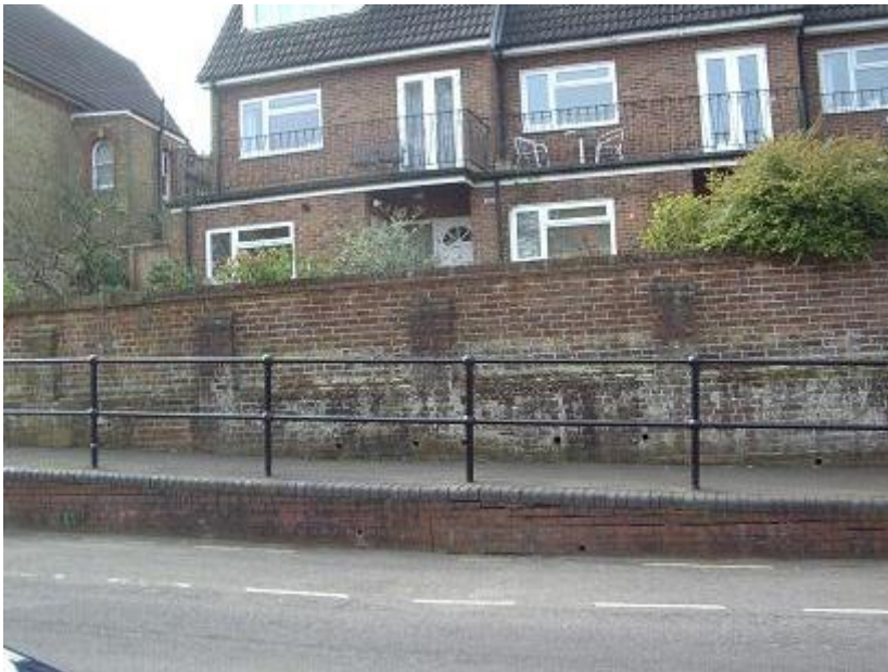
Good new railings on Eardley Road
