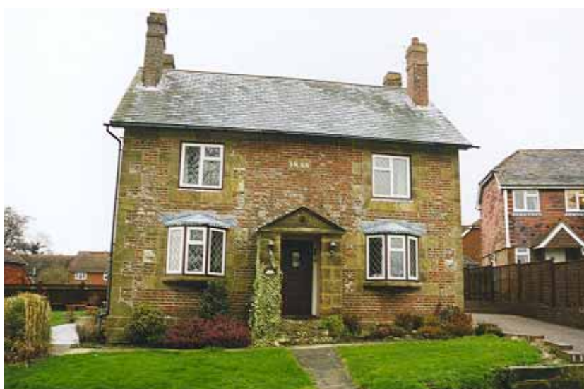
Figure 16 Replacement windows in Bakery Cottage
