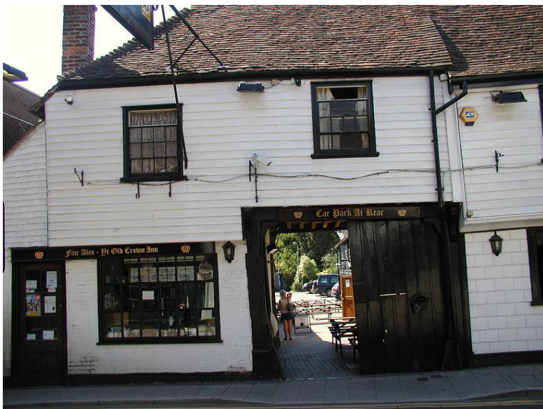
30. White weatherboarding on the Crown Inn (note view through carriage gates)
