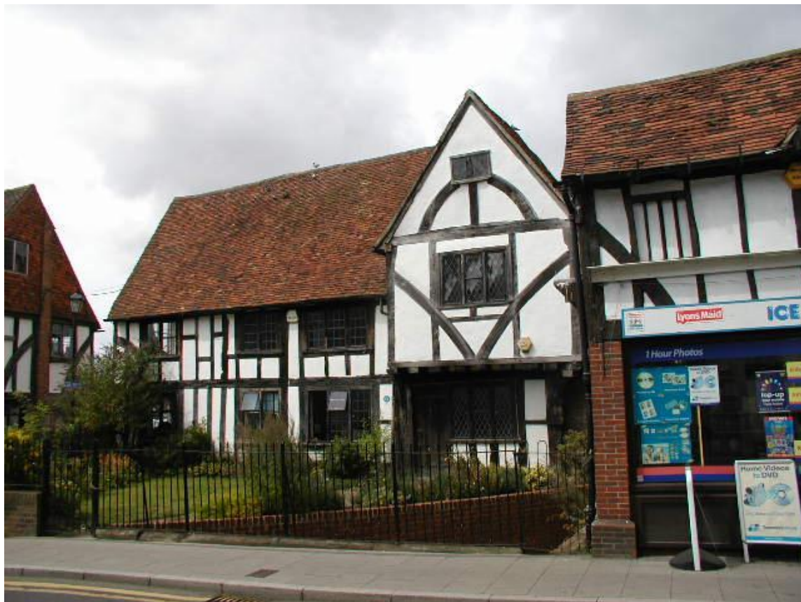
28. Typical Timber Framing to nos. 92 -94 High Street
