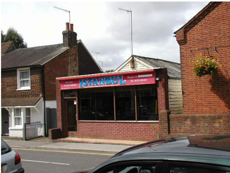
39. Unfortunate shopfront adjoining listed building
