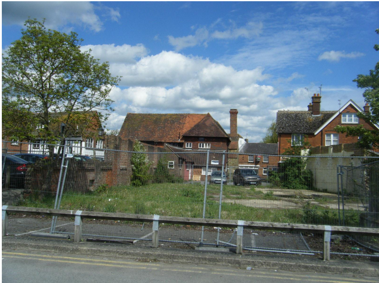
82. This area just behind the High Street should be closely monitored. (there is planning permission for demolition and new flats)
