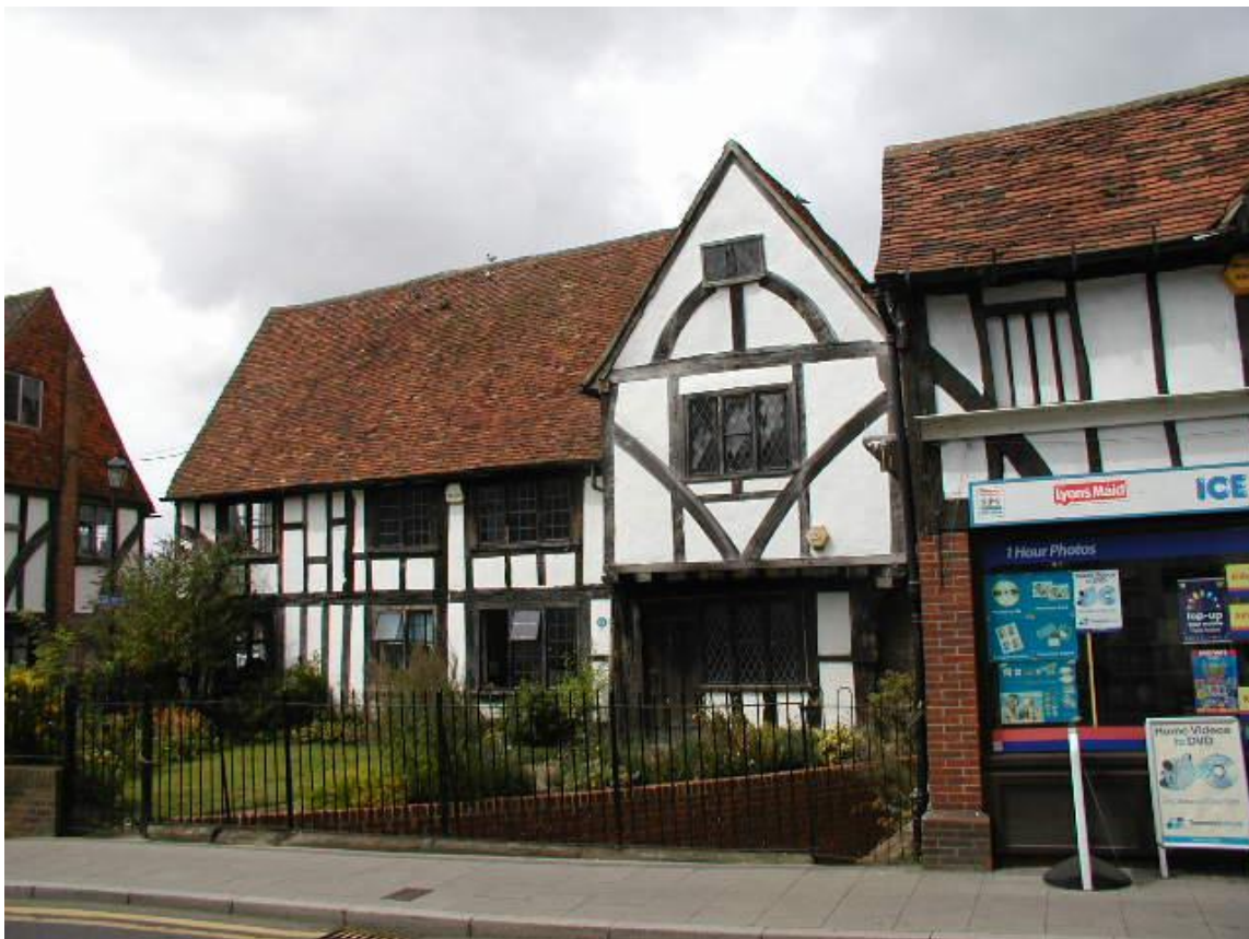
28. Typical Timber Framing to nos. 92 -94 High Street
