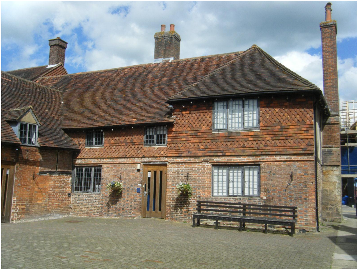
17. Rear view of the fine listed Church House, High Street
