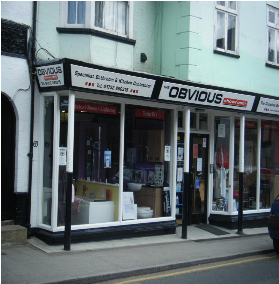
40. A more attractive and distinctive Victorian shopfront
