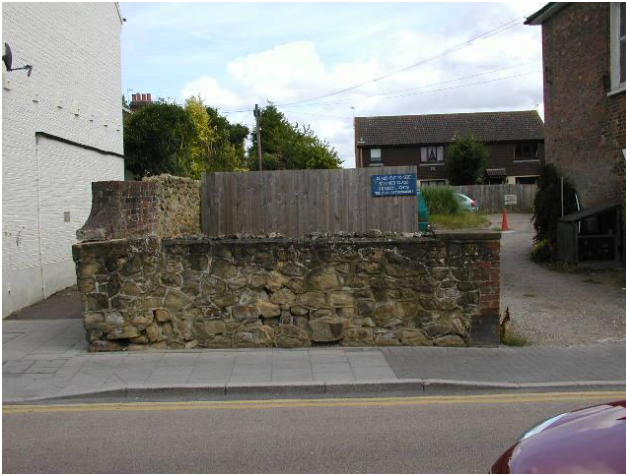
41. Portion of historic wall adjacent to No. 47
