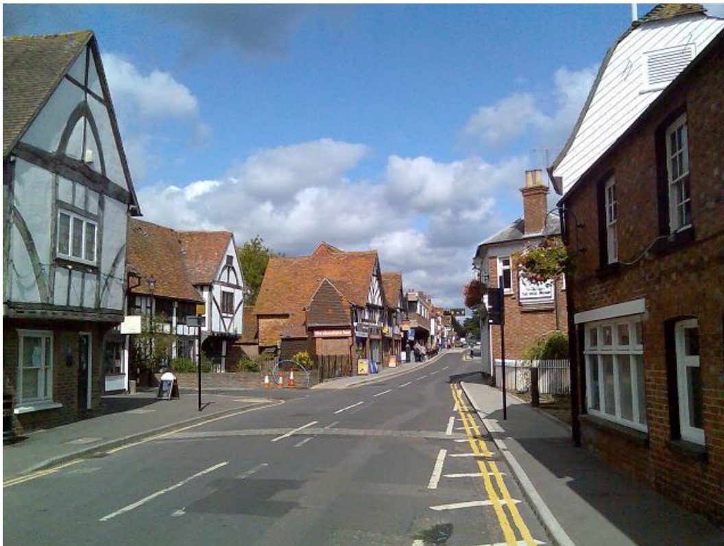
61. Note historic collection of black and white buildings and also some untidy road surfacing.
