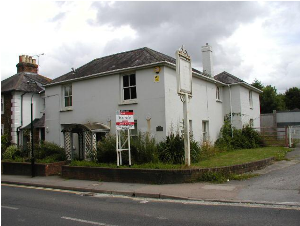
80. This empty historic building in Mill Hill is very prominent and should be monitored
