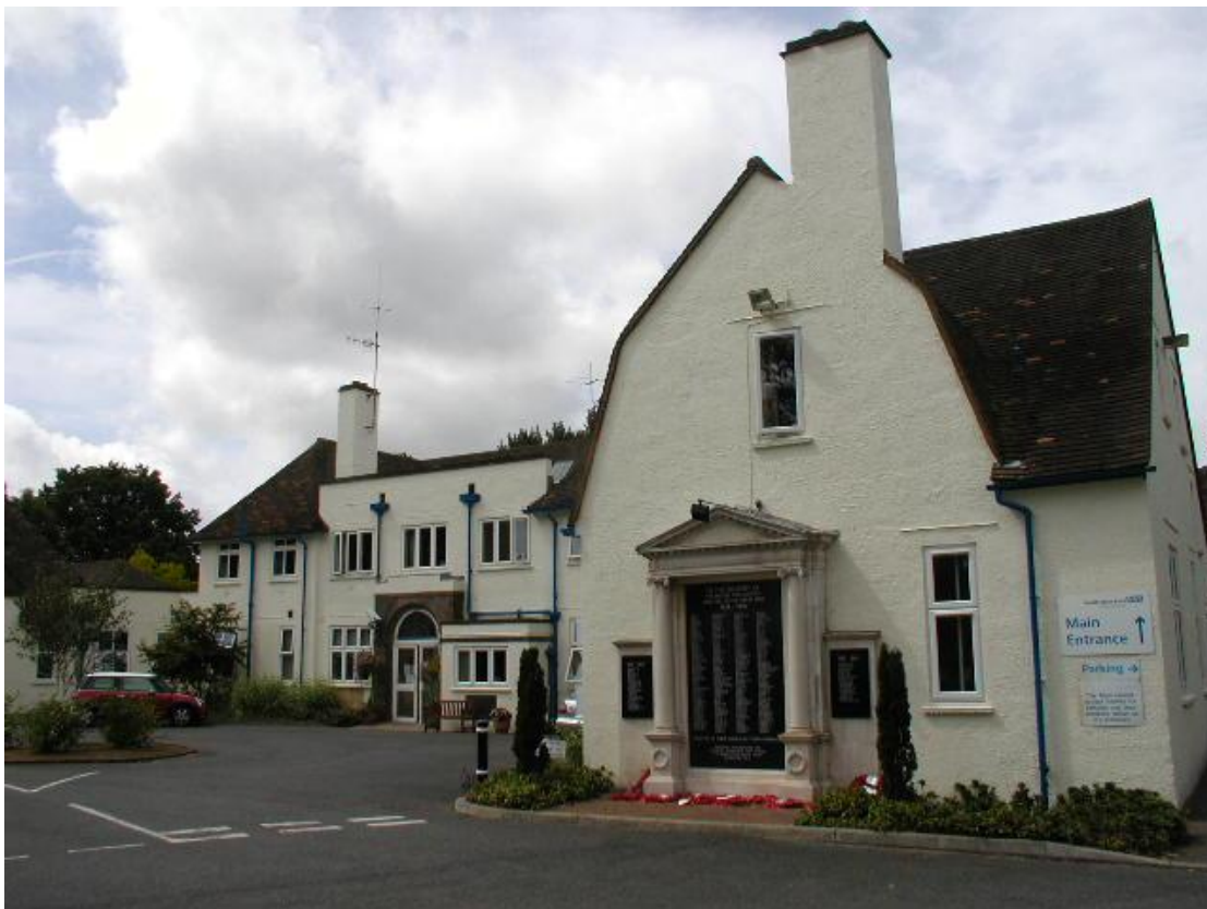
76. This 1930s cottage hospital is suitable in size and scale and of noted historic interest, by Mr H Read of Read and Macdonald, 1928-1931
