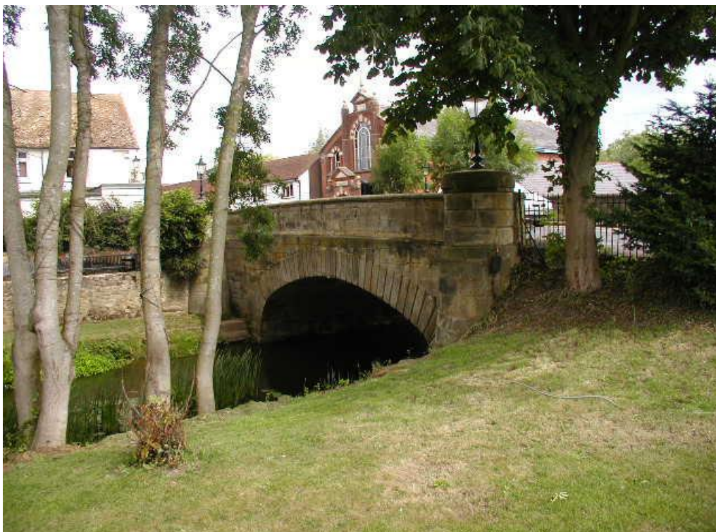
88. The Great Stone Bridge is a key historic feature within the Conservation Area.
