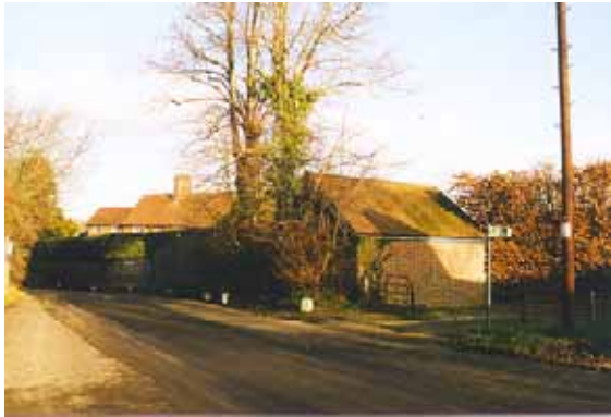
Figure 28 Garage adjacent to The Priors
