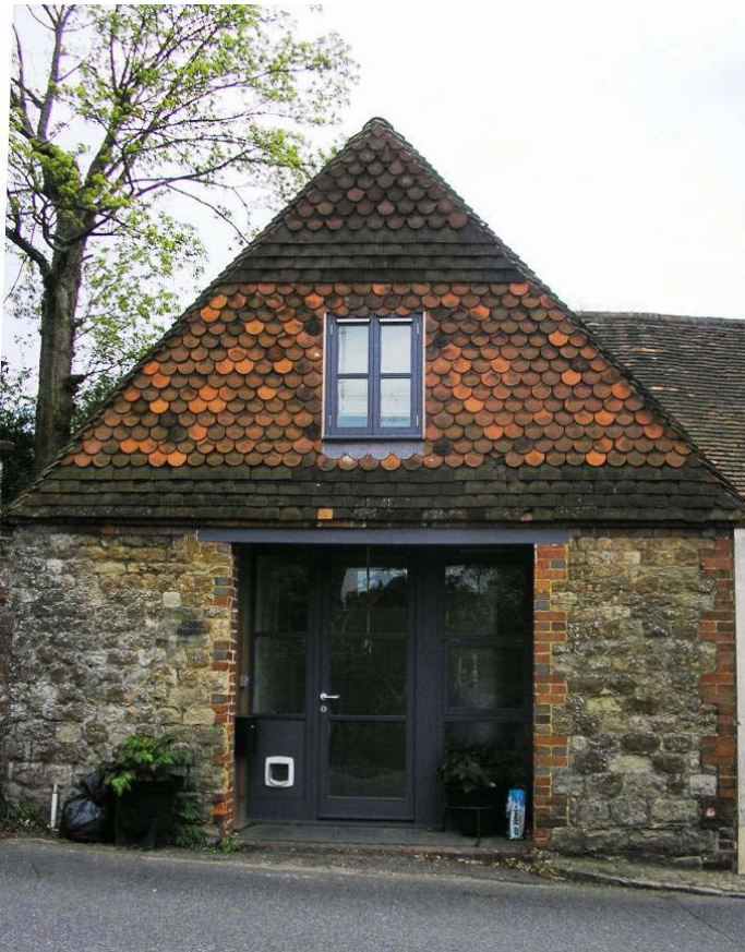
A simple modern conversion retaining original character
