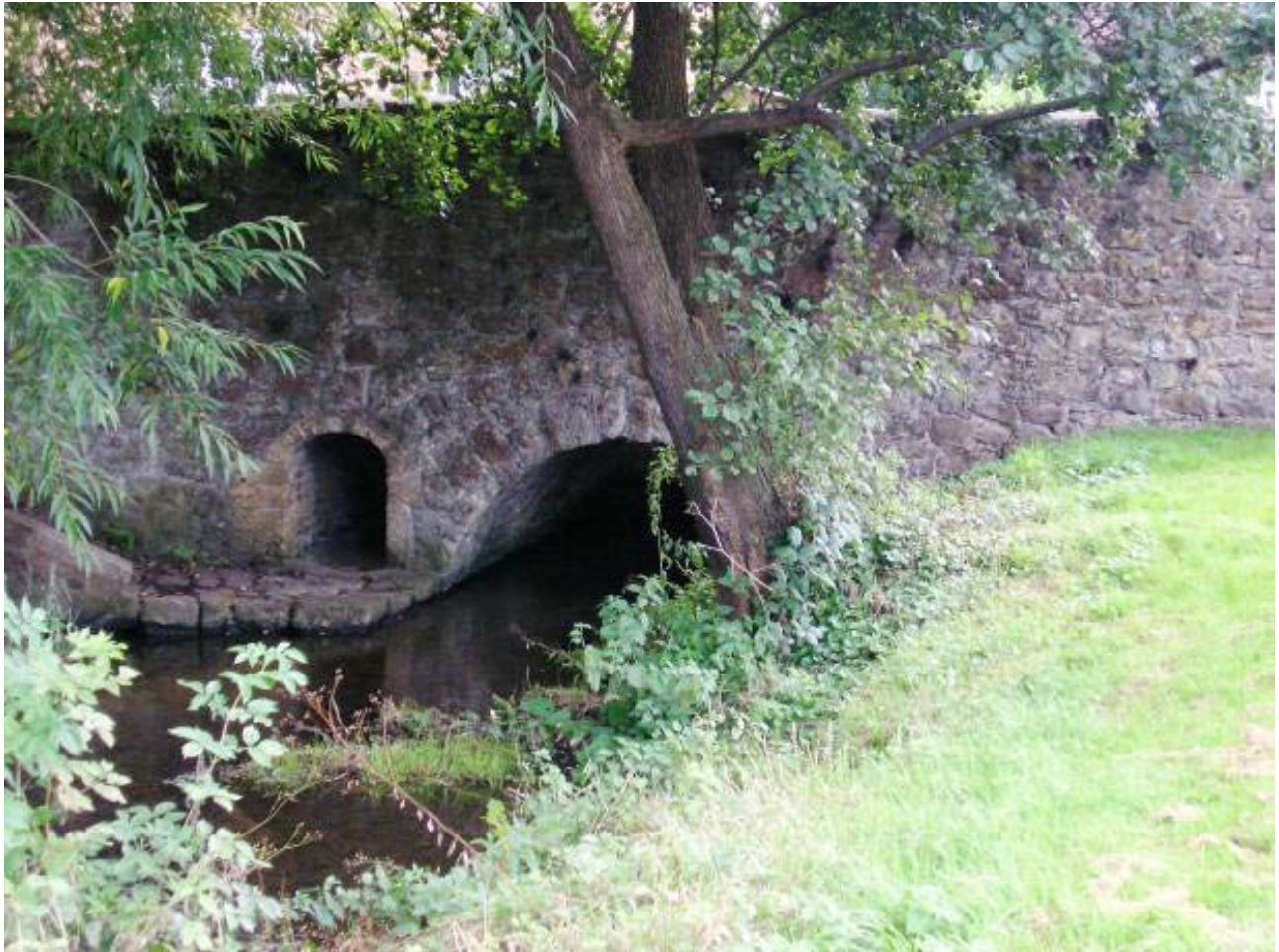
Historic ragstone bridge
