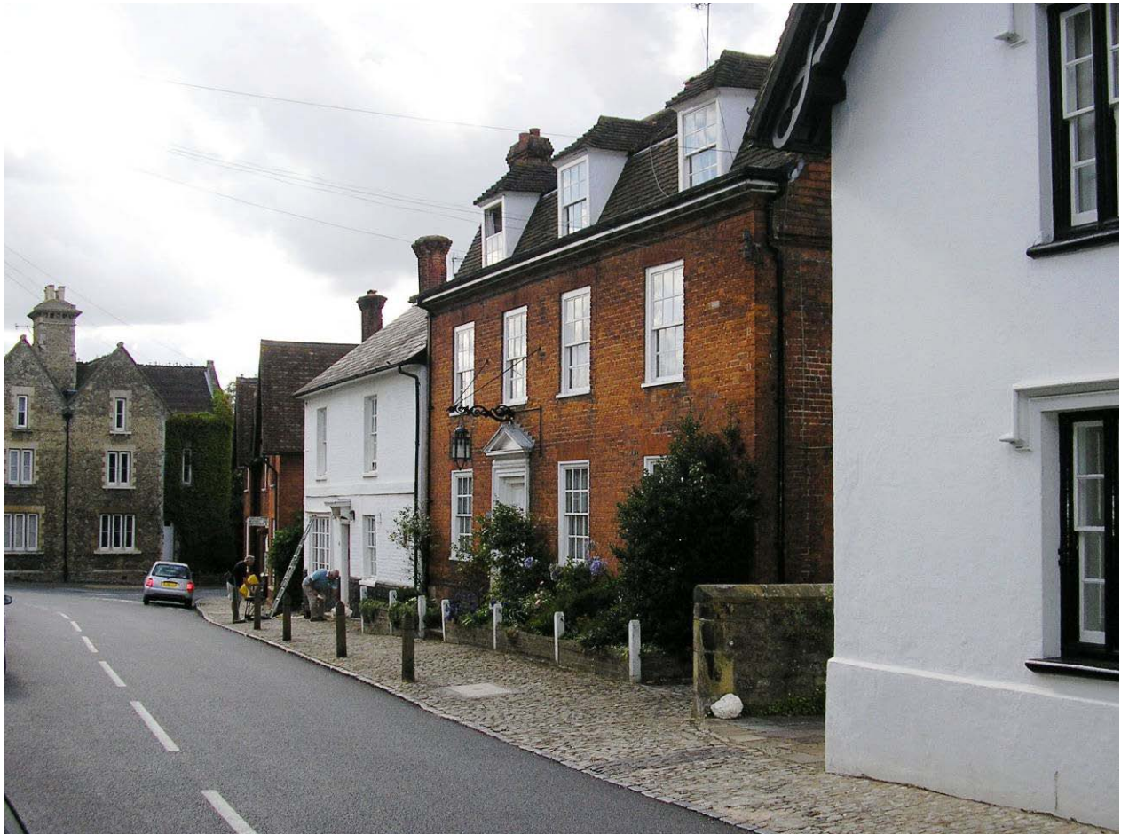
An harmonious mix of building styles including Crown House, formerly an inn.
