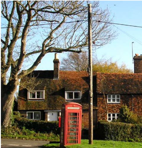
Figure 18 Prominent pole and overhead lines'
