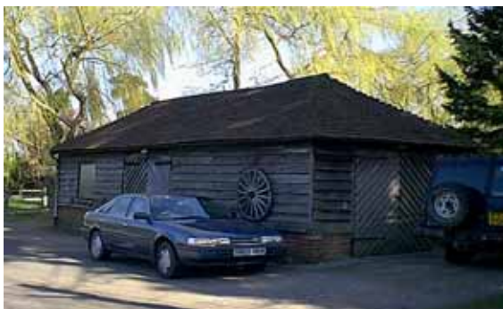
Fig. 59 Timber shiplap outbuilding with Kent peg-tile roof
