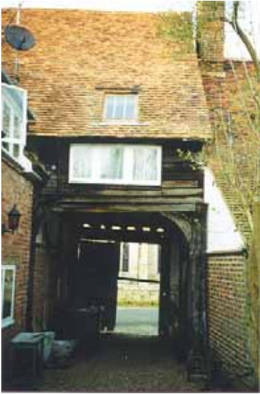
Fig. 33 Rear elevation of Chiddingstone Burghesh Manor
