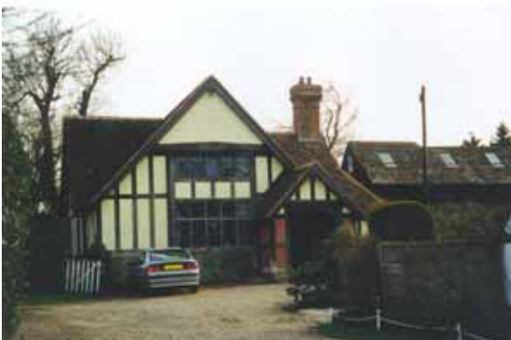
Fig 16 The refurbished Village Hall (former parish room dated 1907 )
