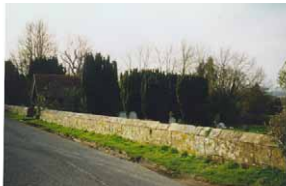
Fig. 30 Boundary wall and lychgate to Cemetery.
