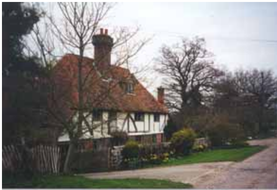
Fig. 52 Wealden House at Hill Hoath
