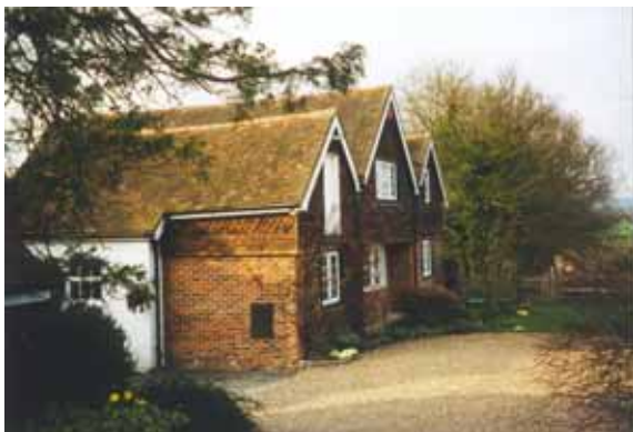
Fig 13 Coachmans with door at first floor level clearly visible
