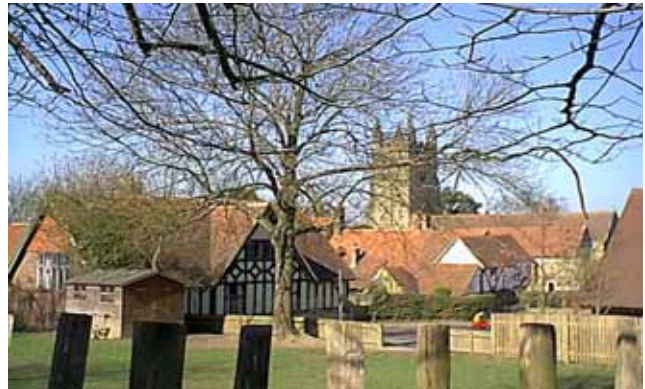
Fig. 19 View looking north west showing Parish Room and the church
