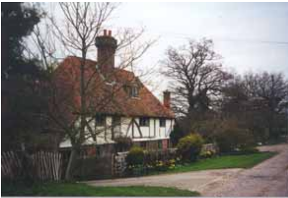
Fig. 52 Wealden House at Hill Hoath
