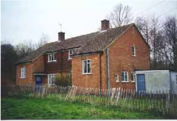
Fig. 60 New houses at Hill Hoath
