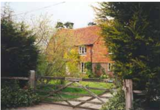
Fig. 54 Hill Hoath House
