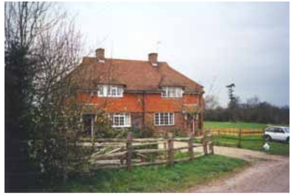
Fig. 56 Hill Hoath Farm Cottages
