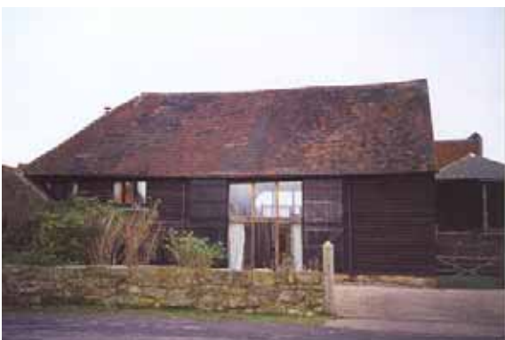
Fig 10 Converted barn adjacent to Larkin's Farm
