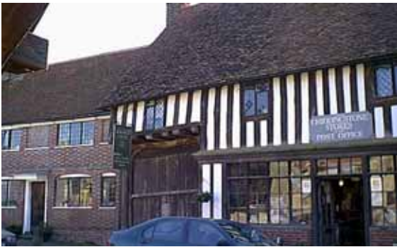
Fig. 22 Chiddingstone Post Office and Shop
