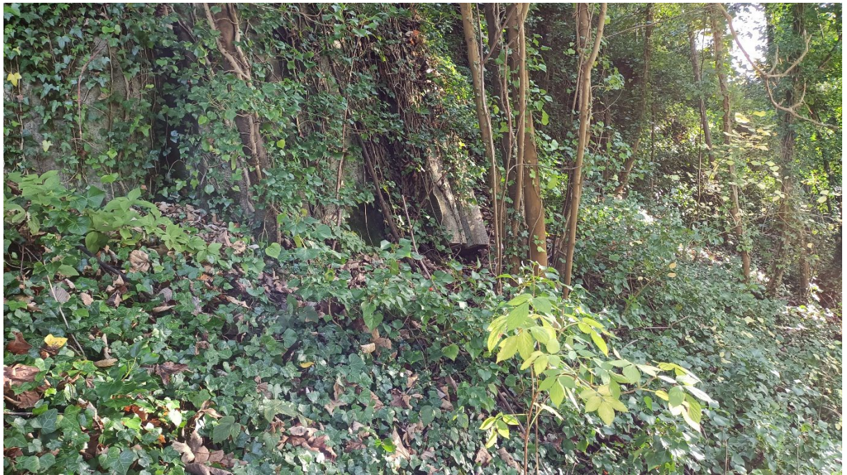
Photo 6 – Concrete piles to wall.
