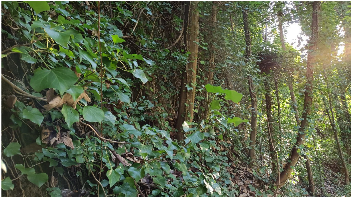
Photo 5 – Vegetation growing on embankment.
