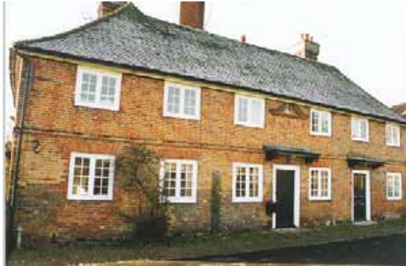
Figure 3 Cottages in Chevening Road
