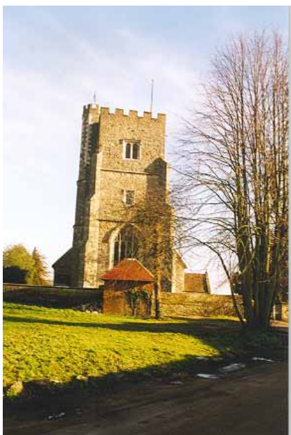
Figure 6 St. Botolph's Church
