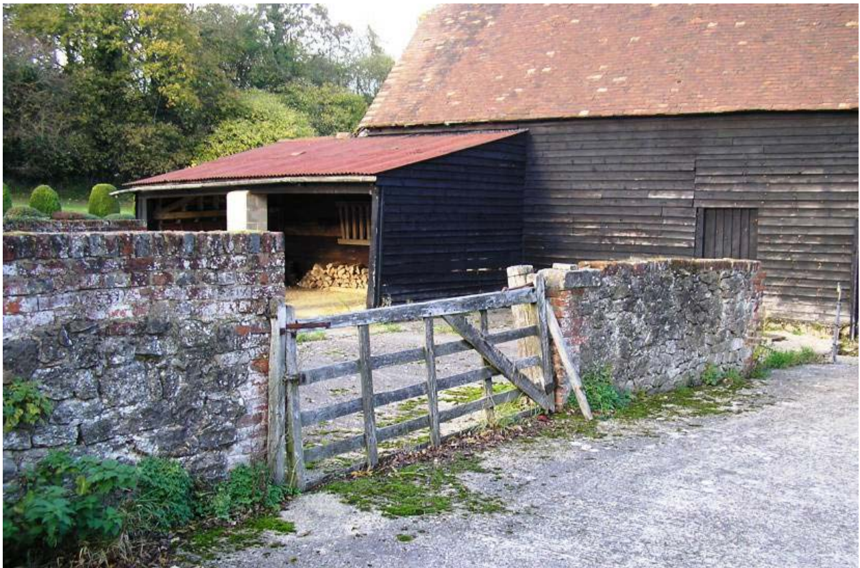
Ragstone and brick wall adds to the character of this farmstead group
