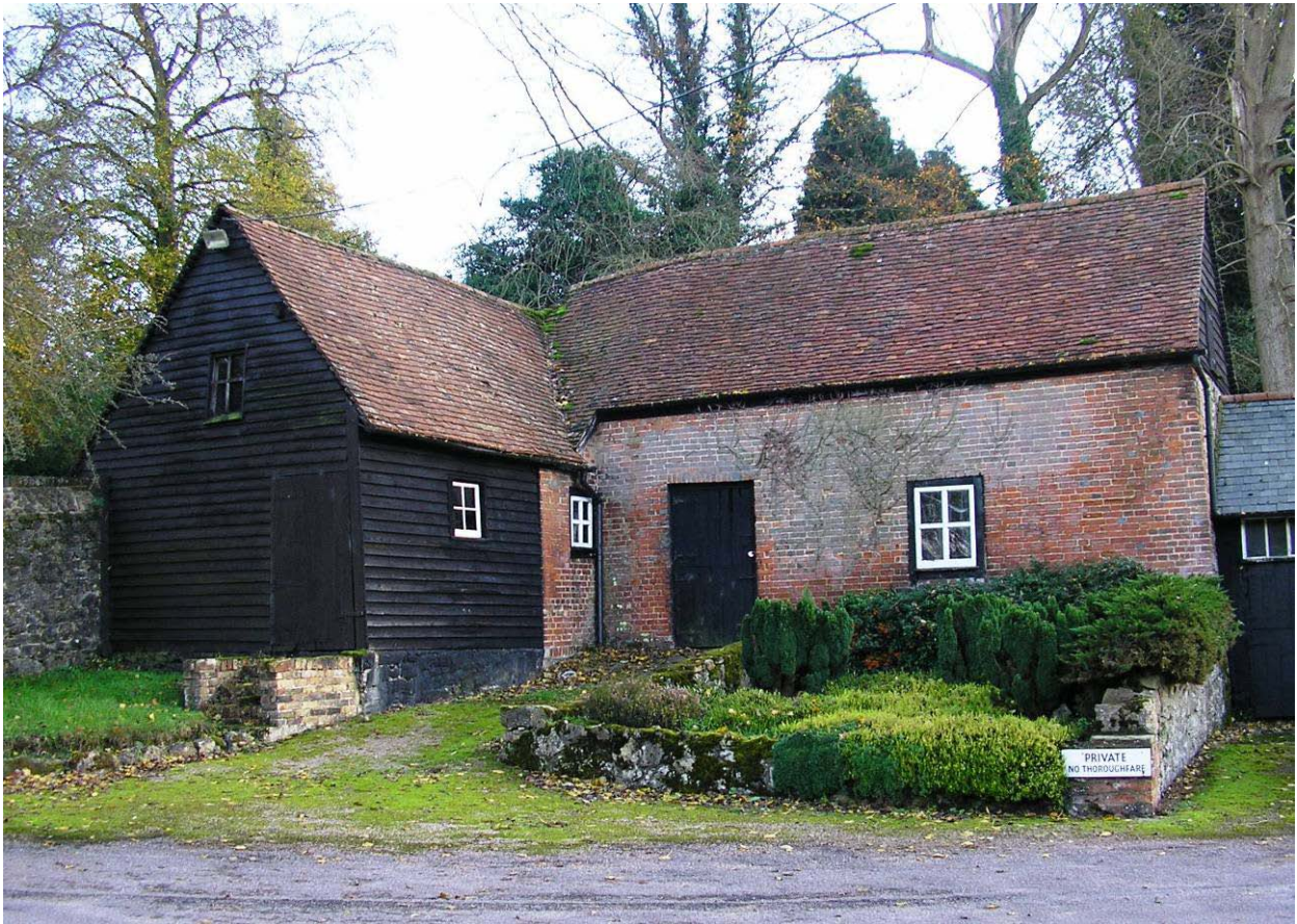
A limited palette of hand made vernacular materials adds to the character of this building.
