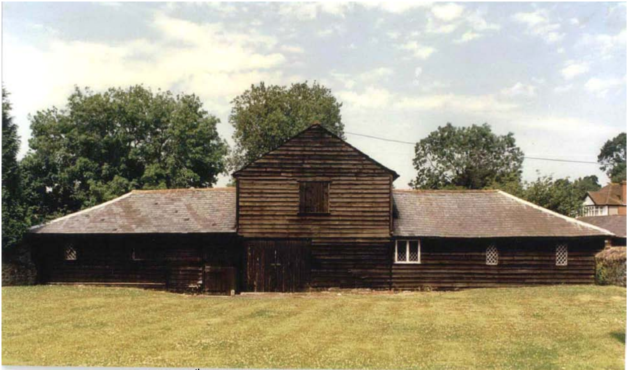
The symmetrical elevation and 19 th Century lattice windows indicate a considered design for this former agricultural building perhaps reflecting its origins as an Estate building
