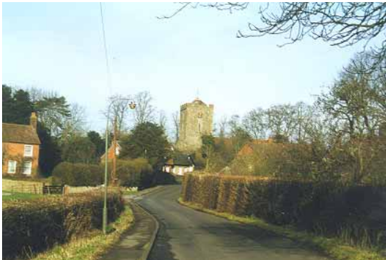
Figure 5 View from the south towards the church
