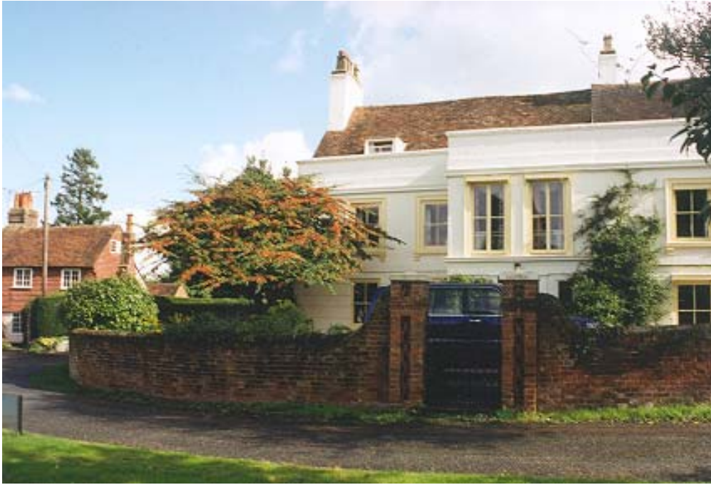
Figure 13 The wall in front of Southdown House
