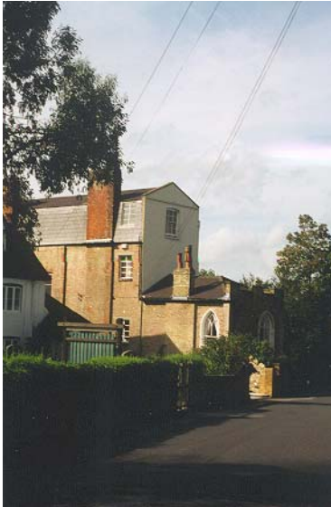
Figure 6 The rear elevation of Bessels House
