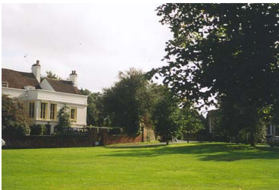
Figure 12 The Green and Southdown House
