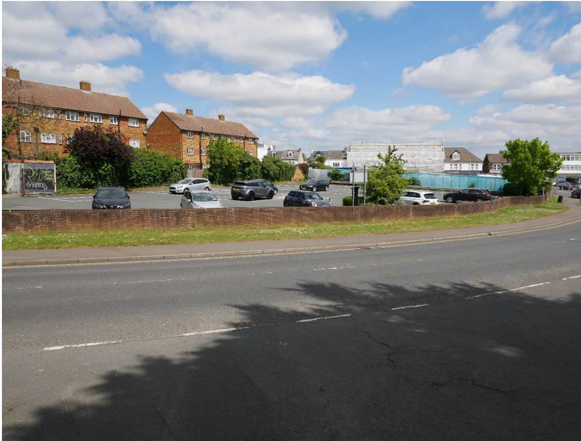
A view of car park CP9 and the hoarding around the demolished old social club. The three-story flats in the back ground (TC24) may be demolished to form part of the new development.
