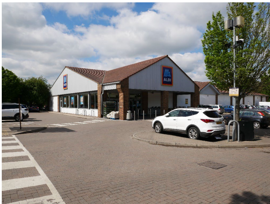
TC10-1 ALDI store showing the designated footway
