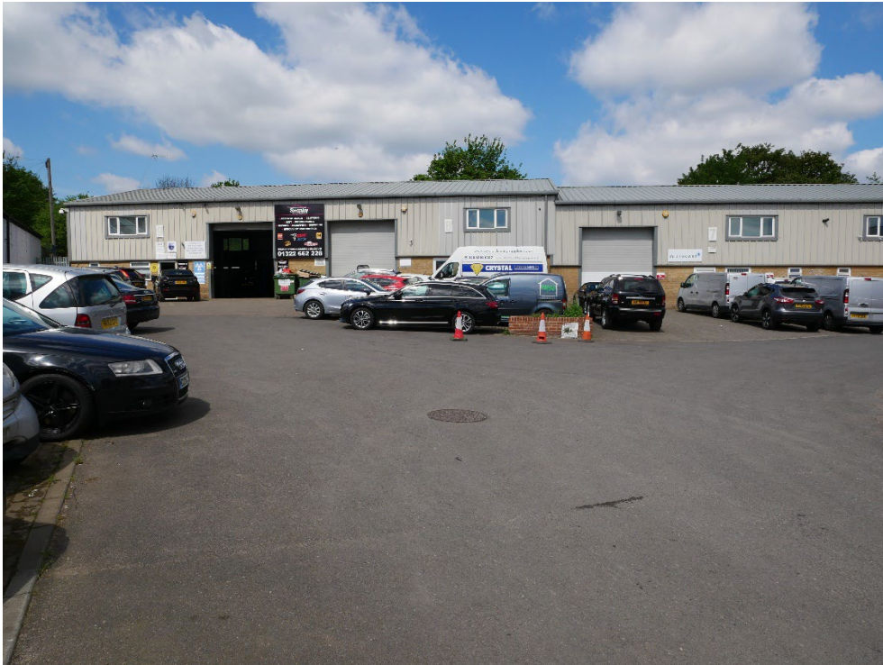
A view of the newer light industrial units at Park Road
