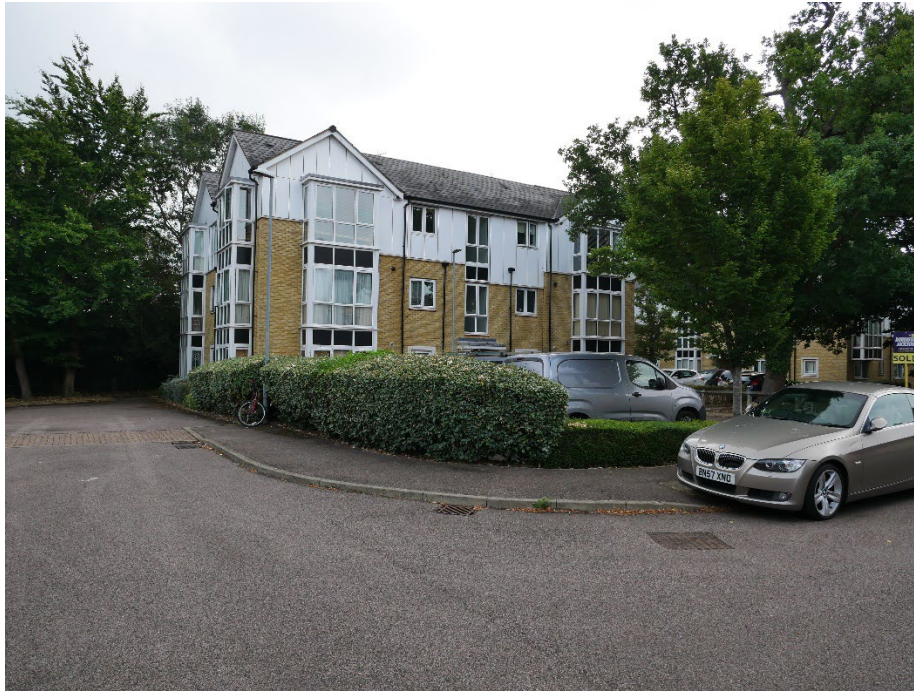
A view of the three-storey private flats in Squirrels Close looking east
