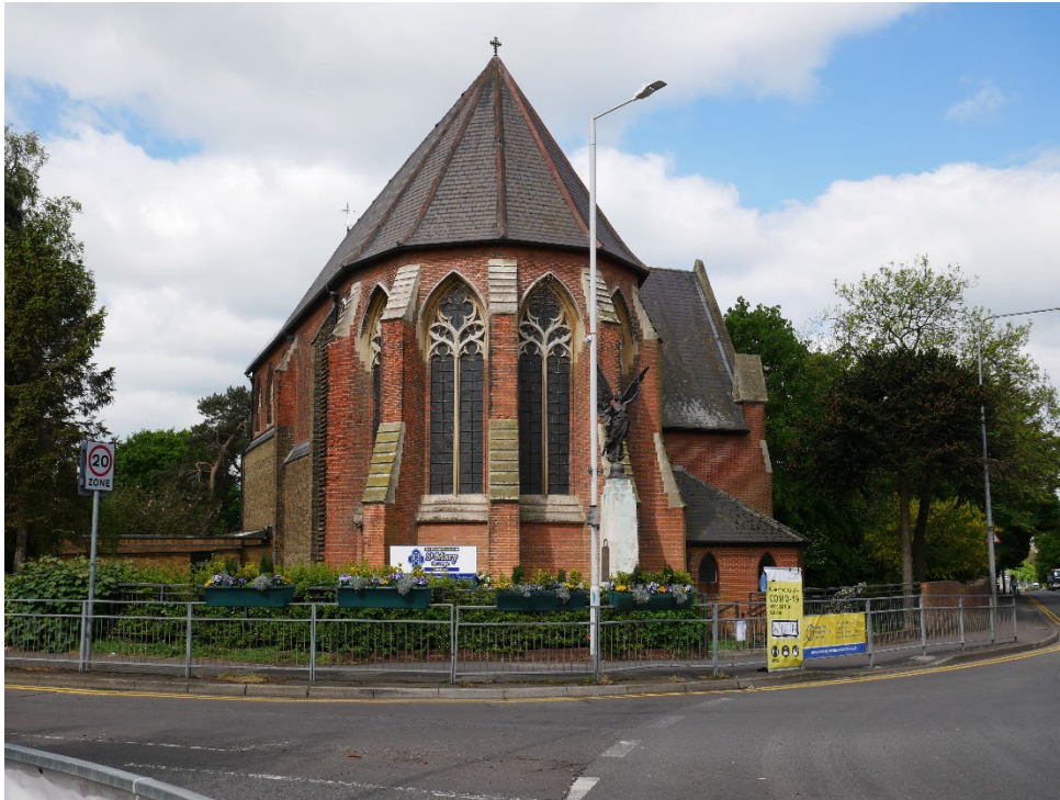
H10 A view of St Mary's Church from the roundabout connecting London Road to Bartholomew Way and St Mary's Road. Note the war memorial to the right of the lamp post which used to be located at the junction of the High Street and Swanley Lane which is now part of ASDA's car park.
