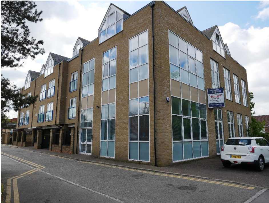
TC14-1 Little Heath viewed from St Mary's Road showing business units at the front and flats to the rear.
