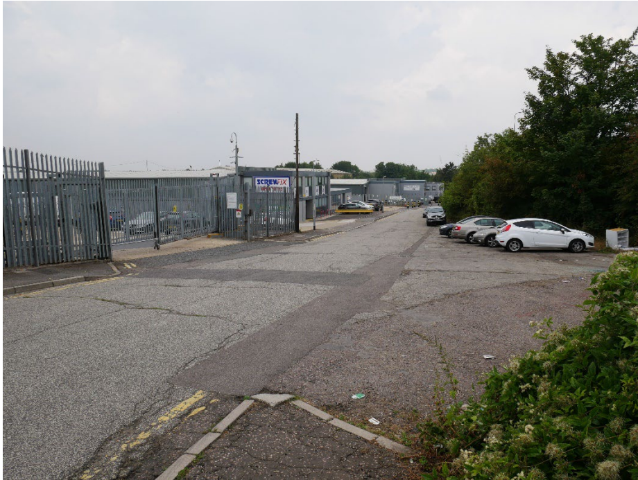
A view of the Mark Way business development from Wested Lane.
