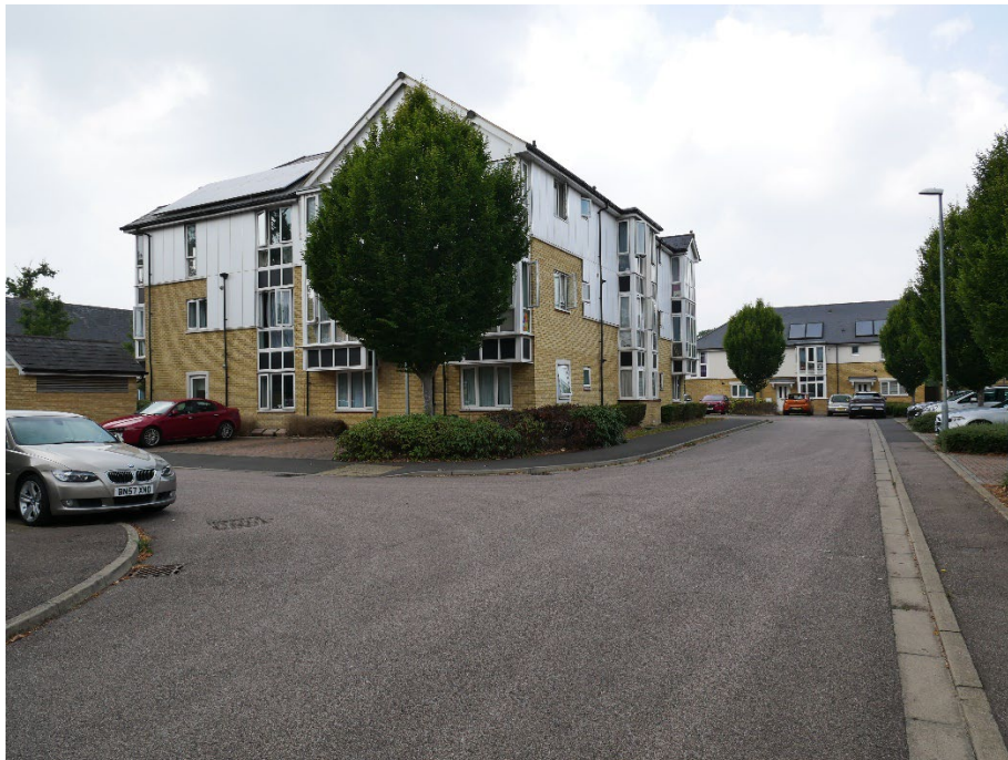
A view of the three-storey private flats in Squirrels Close looking west
