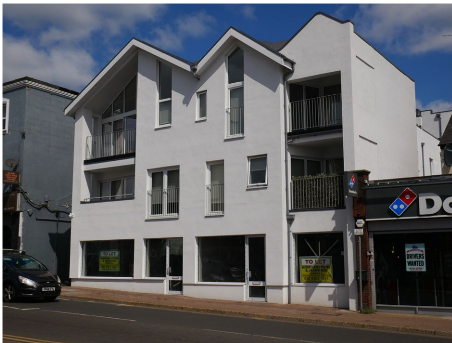
TC27 11-13, High Street view of the new mixed-use development.
