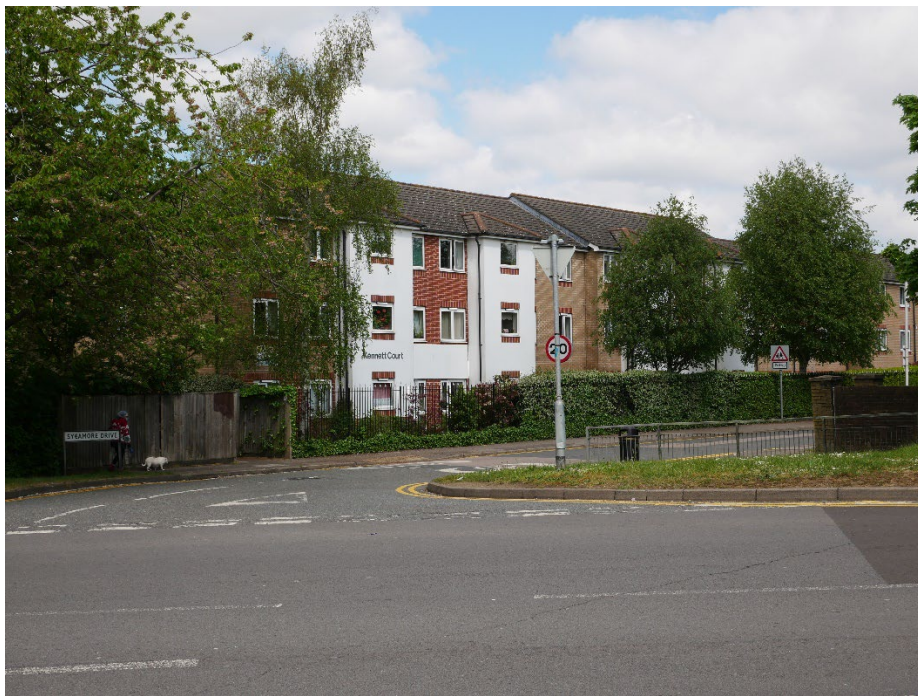
A view of the three-storey private retirement development in Sycamore Drive taken from Bartholomew Way.
