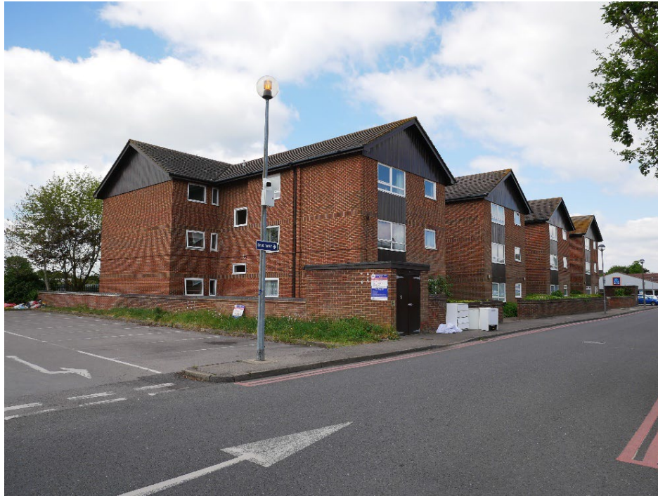
TC12 Berkeley Court residential flats viewed from Nightingale Way. The recreation ground is to the rear.
