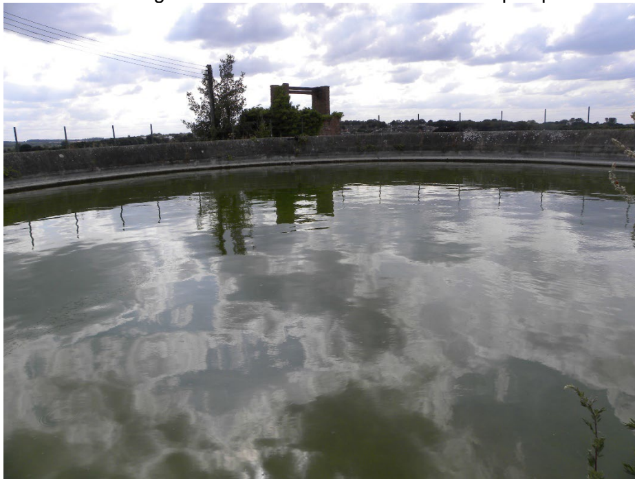
A view inside the Victorian water reservoir.
