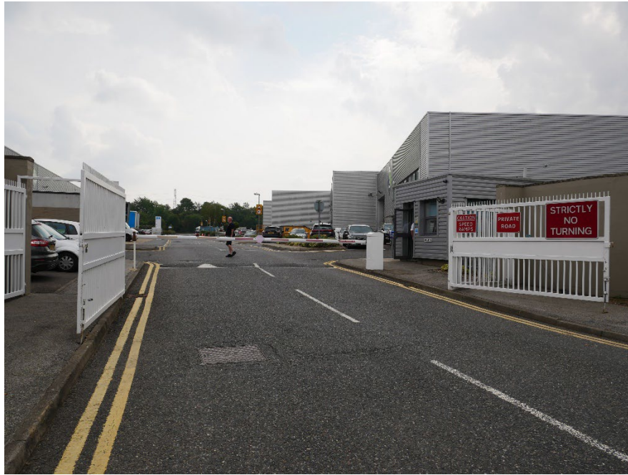
A view of the East side of the Interchange business development from Wested Lane.
