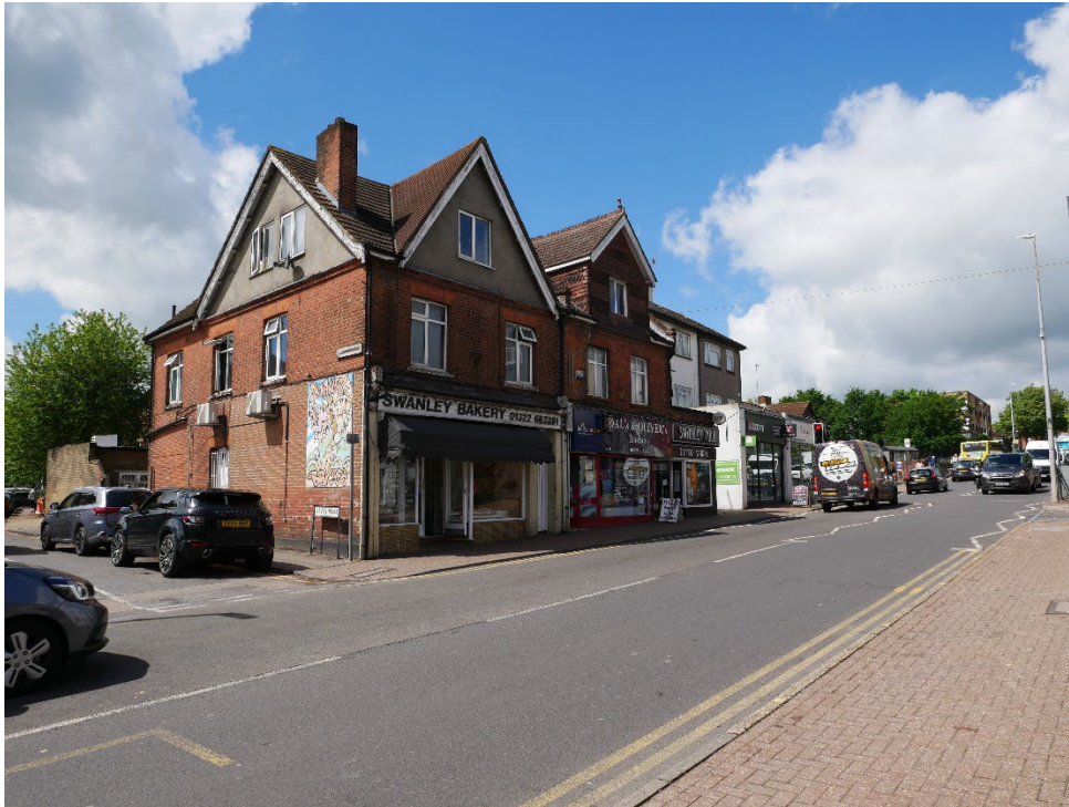
TC21 The South side of the High Street on the corner of Bevan Place Road showing the two storey terraced shop units with roof dormers and three storey units at the far end adjacent to the PH.
