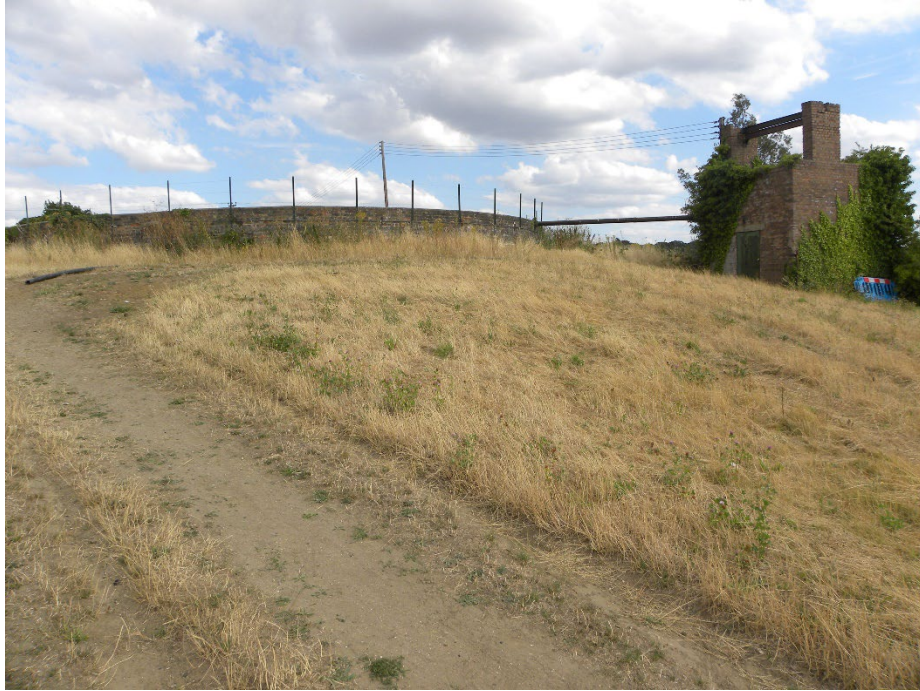
A view showing the Victorian reservoir and bore hole pump house.
