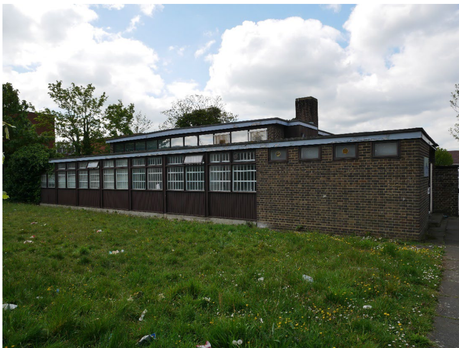
TC17 The telephone exchange viewed from London Road to the left of the fire station.
