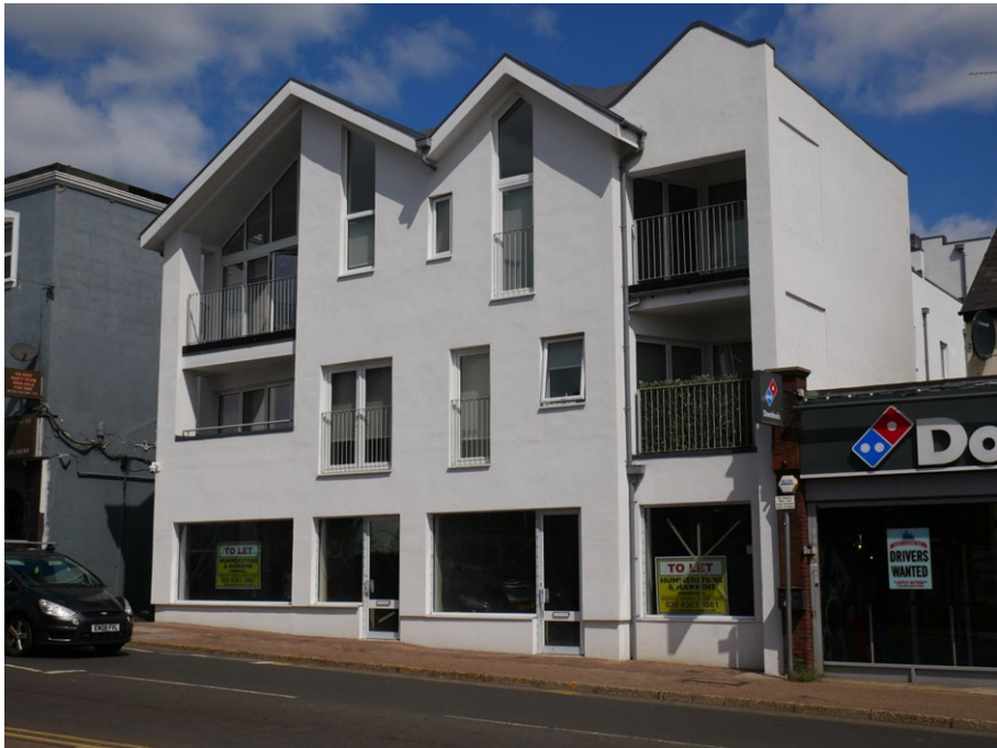
TC27 11-13, High Street view of a new mixed-use development.
