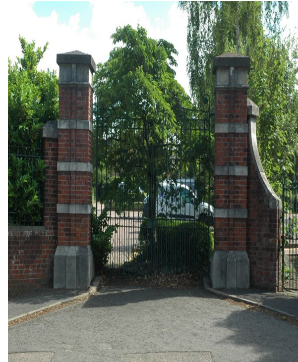
H9 Original main Gateway together with related pillars and short section of the wall (topped in part by iron railings) are all that remain of the former White Oak Hospital (opened 1903, closed 1950).
