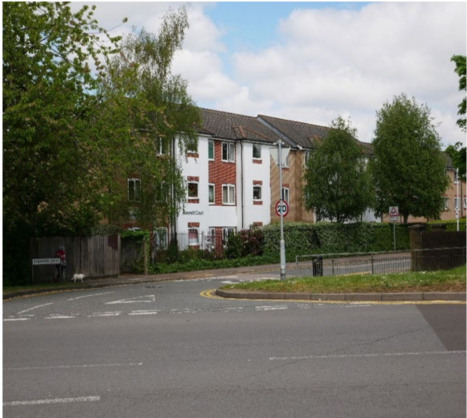
H12 A view of the three-storey private retirement development in Sycamore Drive taken from Bartholomew Way.
