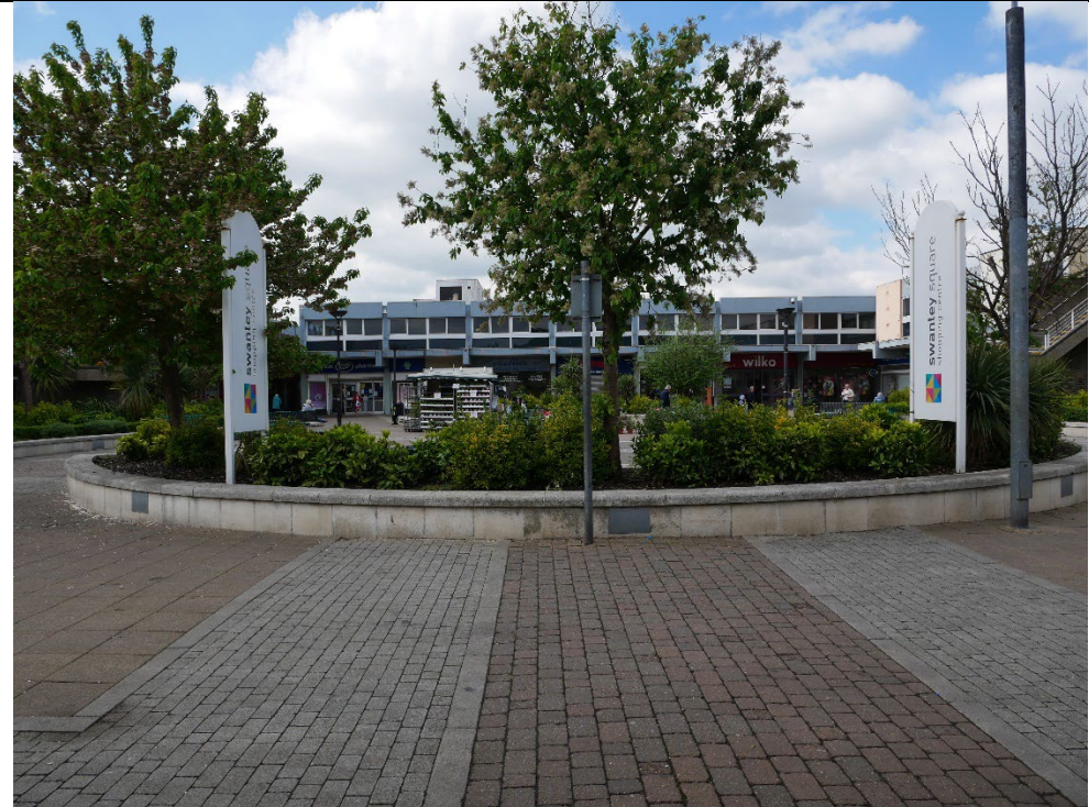
TC5 View of Town Centre 1970's shopping centre into the Town Square from the pedestrianized London Road
