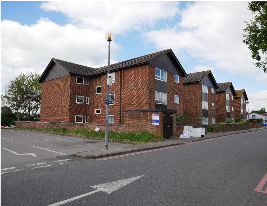
TC12 Berkeley Court residential flats viewed from Nightingale Way. The recreation ground is to the rear.
