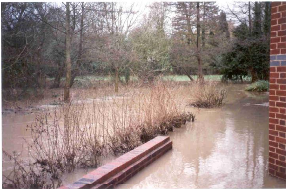
Photo: Property flooding in Brasted December 2002
