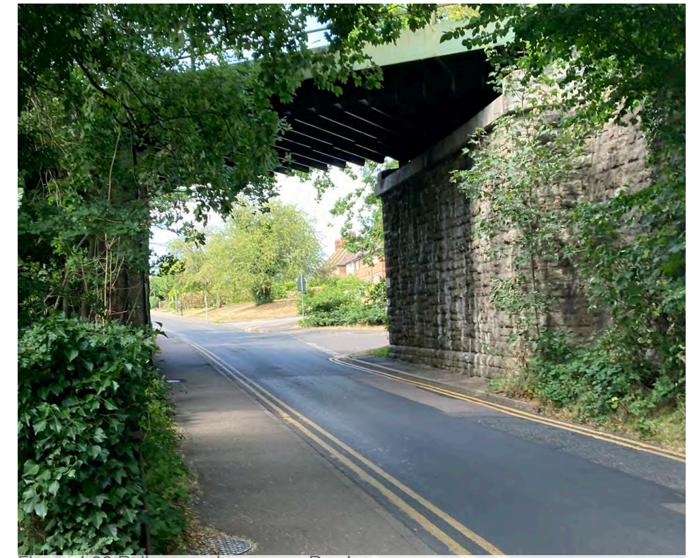
Figure 4.20 Railway underpass on Rye Lane
