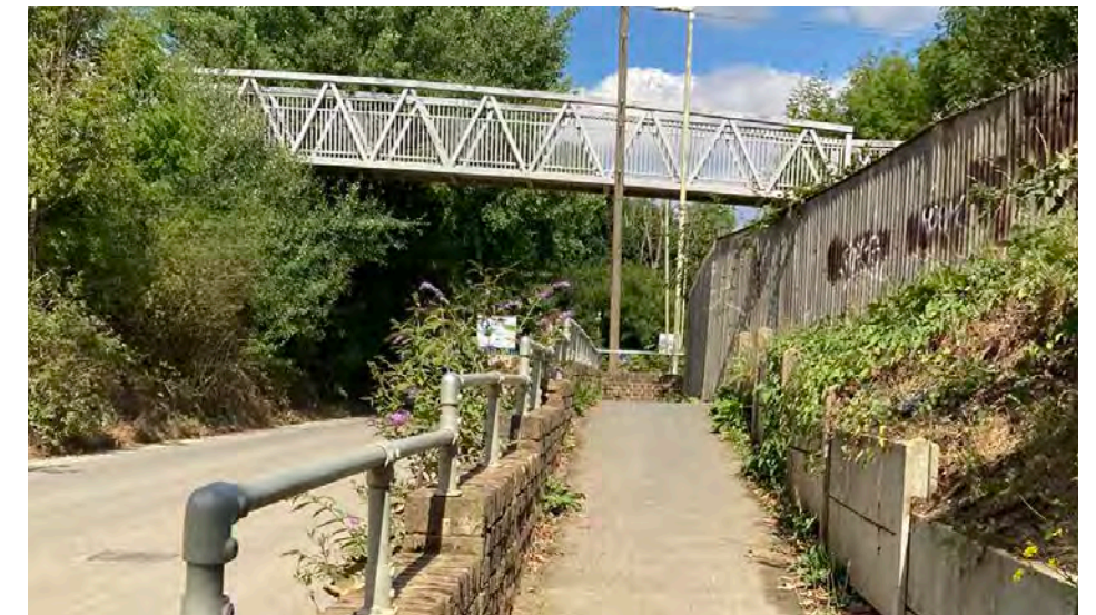
Figure 4.31 Existing footbridge over Bat and Ball Road
