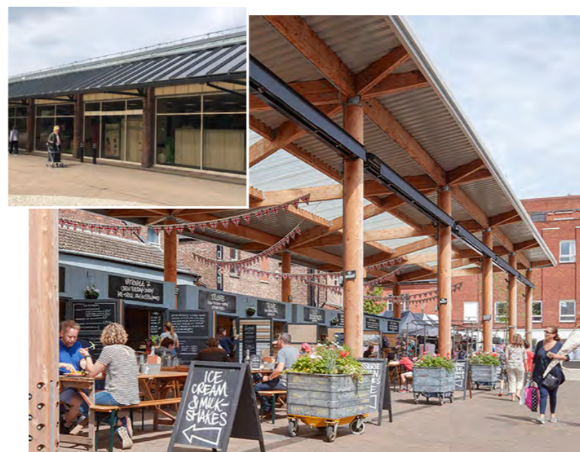
Central Way, Altrincham. Project to provide a new market canopy for market stalls and seating, with associated public realm upgrades to materials, lighting, and planting. The project has helped to extend market activities beyond the adjacent market hall into the surrounding streets. This type of intervention could be appropriate to Asda Walk to both support market activities and animate blank walls.
