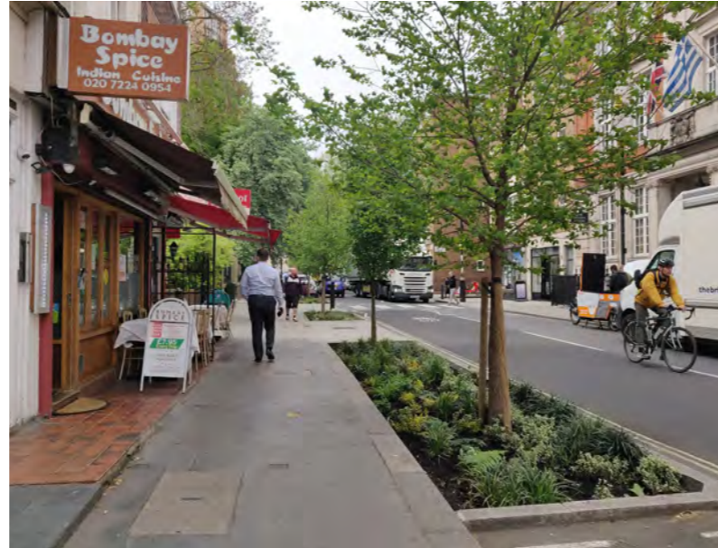
Case Study: Marylebone Low Emission Neighbourhood. Integrated rain gardens and street trees, frequent pedestrian crossings, carriageway narrowing, and reduced turning radii to side streets collectively work to reduce vehicle speeds, maximise space for pedestrians, and improve air quality along the high street. ©Urban Movement
