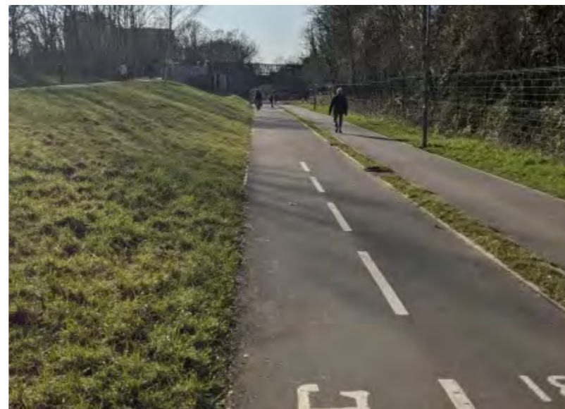
Beeline cycleway in Kingston - a popular and high-quality cycling and walking route alongside a railway. The route is away from main roads, meaning a reduced air and noise pollution. In 2021, sensor data showed, on average, 542 cyclists and 703 people walking used the route each day. ©Kingston Cycling Campaign
