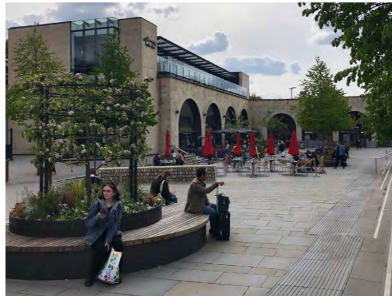
Case study: Bath Station where the Station forecourt has been transformed into a public and green space, providing a positive sense of arrival and improved accessibility. This was achieved through redistribution of car traffic and bus provision, de-cluttering, the introduction of greenery and new active ground floor uses.
