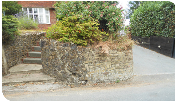
Stone and brick retaining wall
