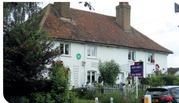
Unbroken roof slopes
