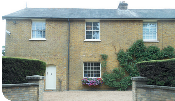
Yellow brick and slate roofs
