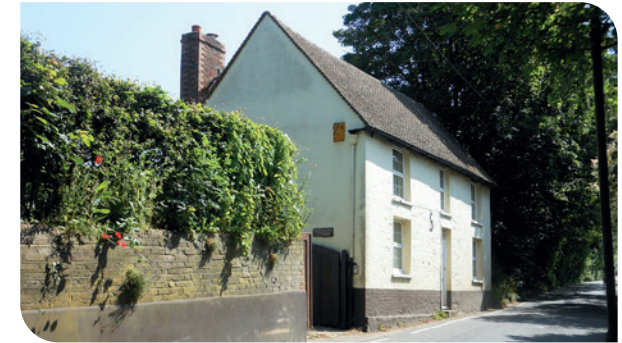
Unbroken roof slopes
