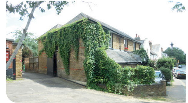
Yellow brick and slate roofs
