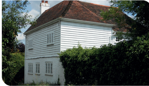
Weatherboarding and brick covering timber frame
