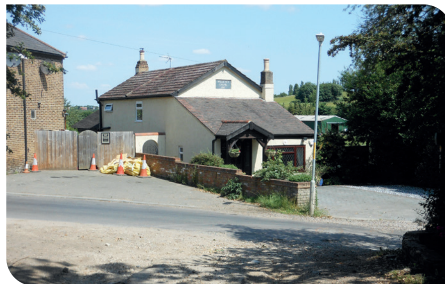
Lack of front boundaries detracts from the character of the conservation area
