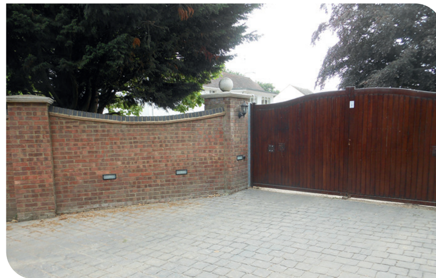
Modern boundary treatment of inappropriate suburban character
