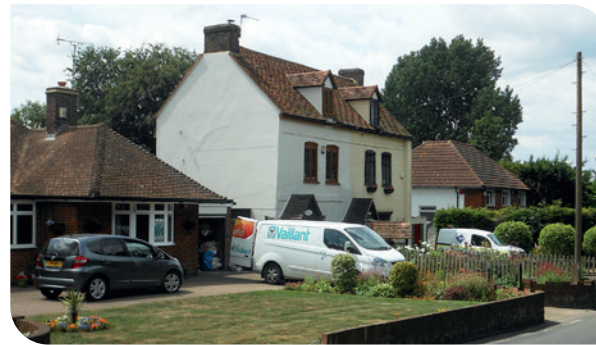
Varied size of building
