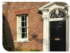
Flemish bond brickwork
