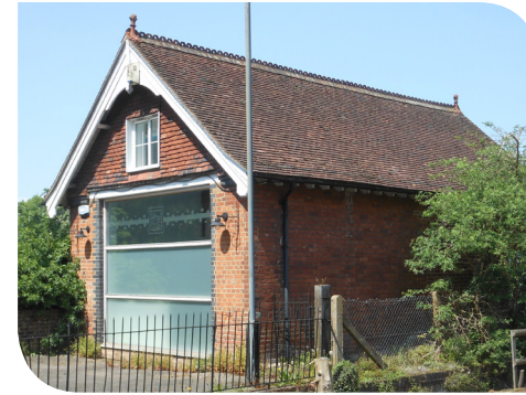
Clay tile roofs with decorative ridges
