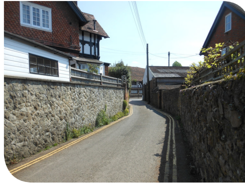
Kentish Ragstone walls
