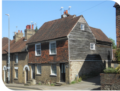
Tile-hanging and weatherboarding
