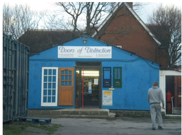
B.6 Doors of Distinction unit on the eastern edge of the site
