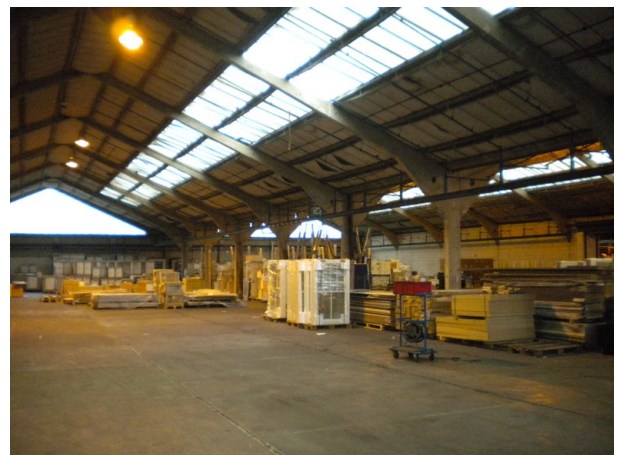
A.6 Inside the main warehouse
