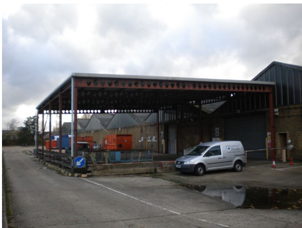
A.5 Eastern side of the main warehouse
