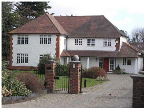
Good Example of an Extended House Ash Rd
