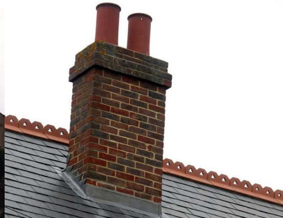
Brick Chimney, Ash Road
