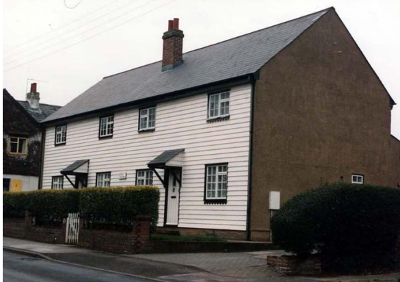
Weather Boarding, Ash Road
