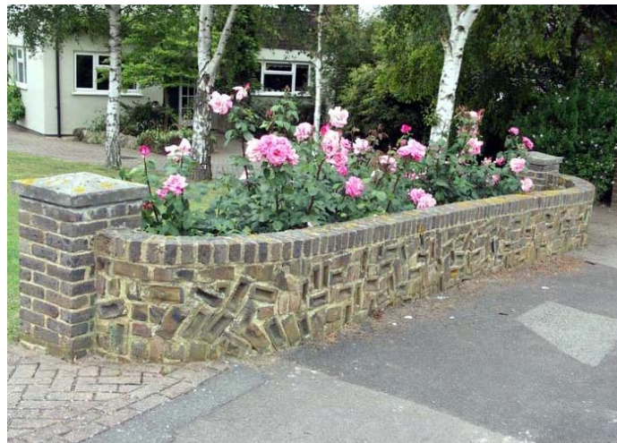
Boundary Wall, Banckside
