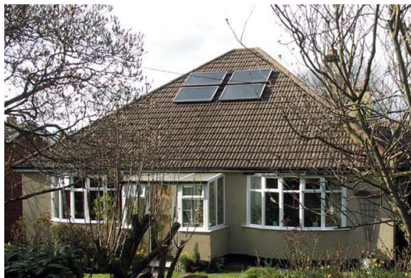
Solar Panels, Stack Lane
