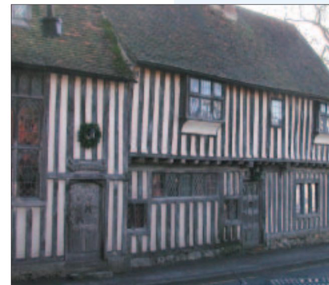
▲ Wattle & daub on a timber frame. Though altered, this oak-framed building is one of Otford's earliest High Street properties.
