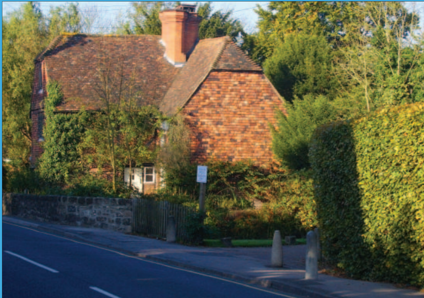
▲ Traditional Wealden farmhouse. The warm colouration of locally made brick with tile-hung façade beneath a barn hip roof of hand-made Kent peg tiles. A typical Kentish yeoman's home.
