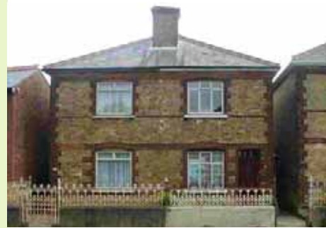
Alma Cottages, Station Road
