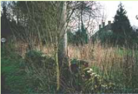
Derelict flint wall in Church Road
