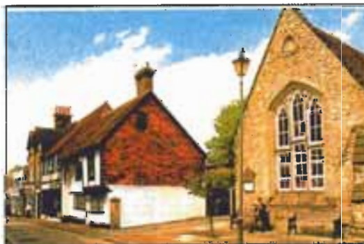
Church Street with the Library. Formerly a school, on the site of the Poor House, and before that The Chequer Inn. Also the early 15thC 'Wealden' called The Priest House.
