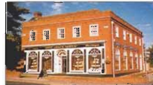
Way Back When Striking & effective renovation of early 20thC building.
