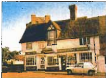
The Square - Eastern Side A single building which was originally a 15thC hall house of a type known as 'Wealden'. It encompasses three shop fronts. The central part with the large dormer window was once the fire station.
