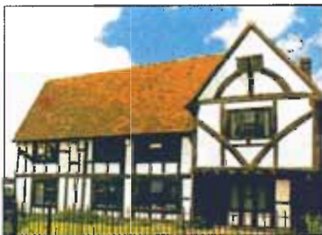
Leather House Formerly Tanyard House. Built with a Cross wing jettied to the north, and East, in the early 15thC. Note the dragon post (a structural method of supporting a double jetty).
