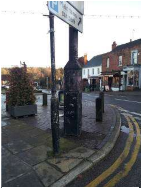
Street furniture in need of maintenance
