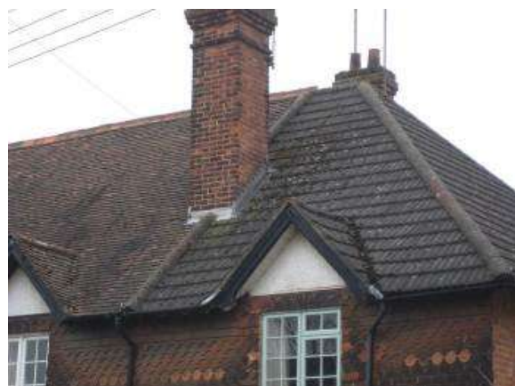
Replacement windows and concrete roof tiles
