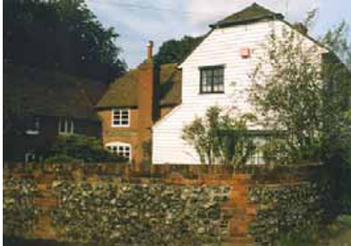
Figure 2 Timber weatherboarding and mellow brickwork on Old College
